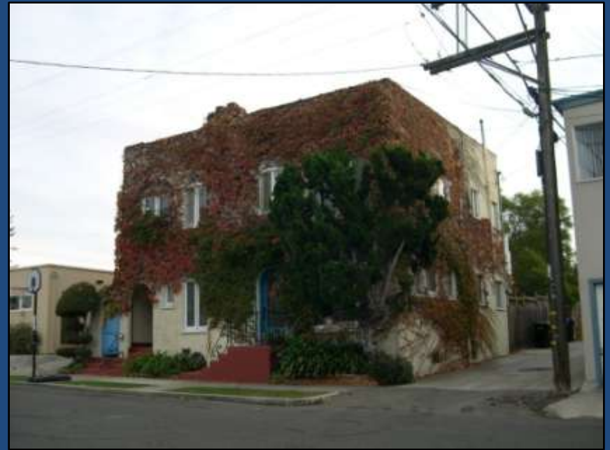
Duplex at 1209 W. Montecito Way
