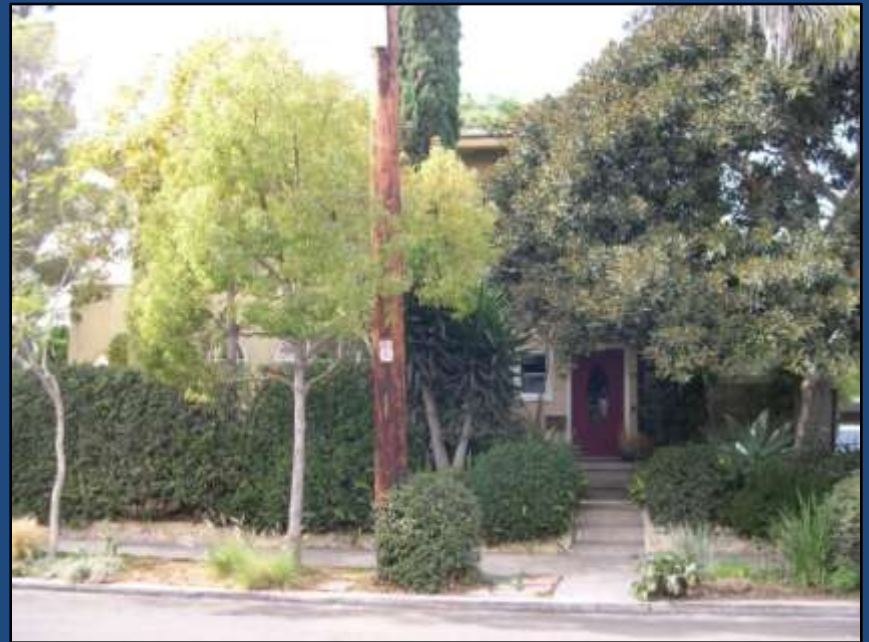
Red side door to second floor unit at 4154 Stephens Street
