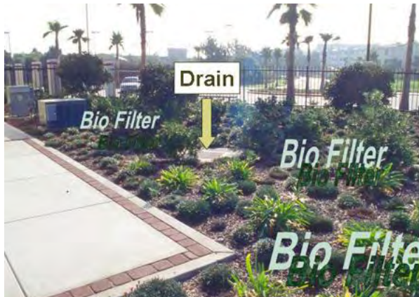
Planted areas and grass swales can serve to treat adjacent impervious areas.
