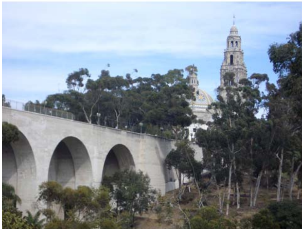
Cabrillo Bridge and Balboa Park
