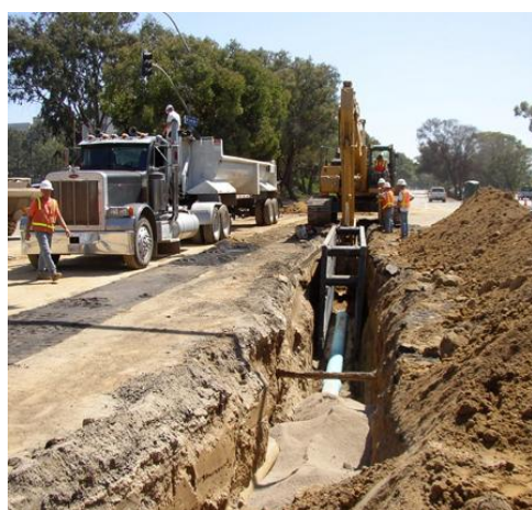
Trenching the municipal sewer system
