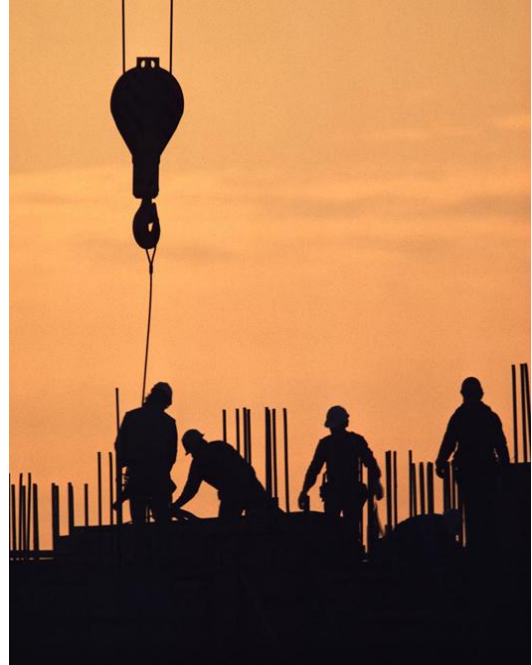
Capital improvements under construction
