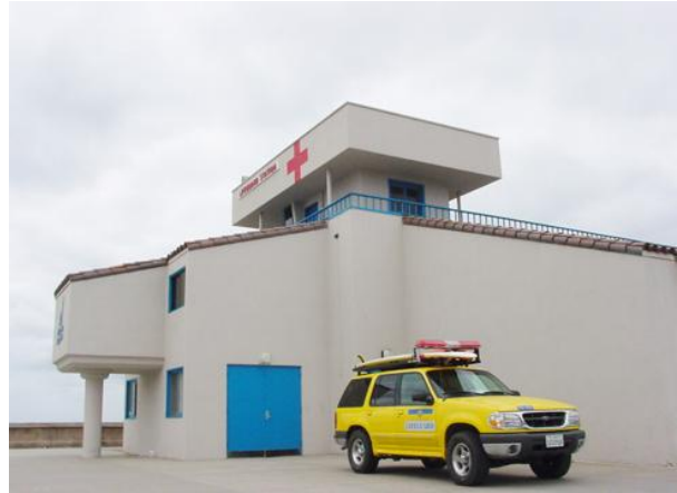
Fire-Rescue Mission Beach Lifeguard Station
