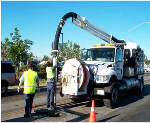
Maintaining the municipal sewer system
