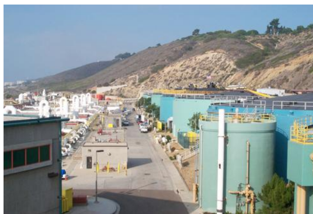
Point Loma Wastewater Treatment Plant
