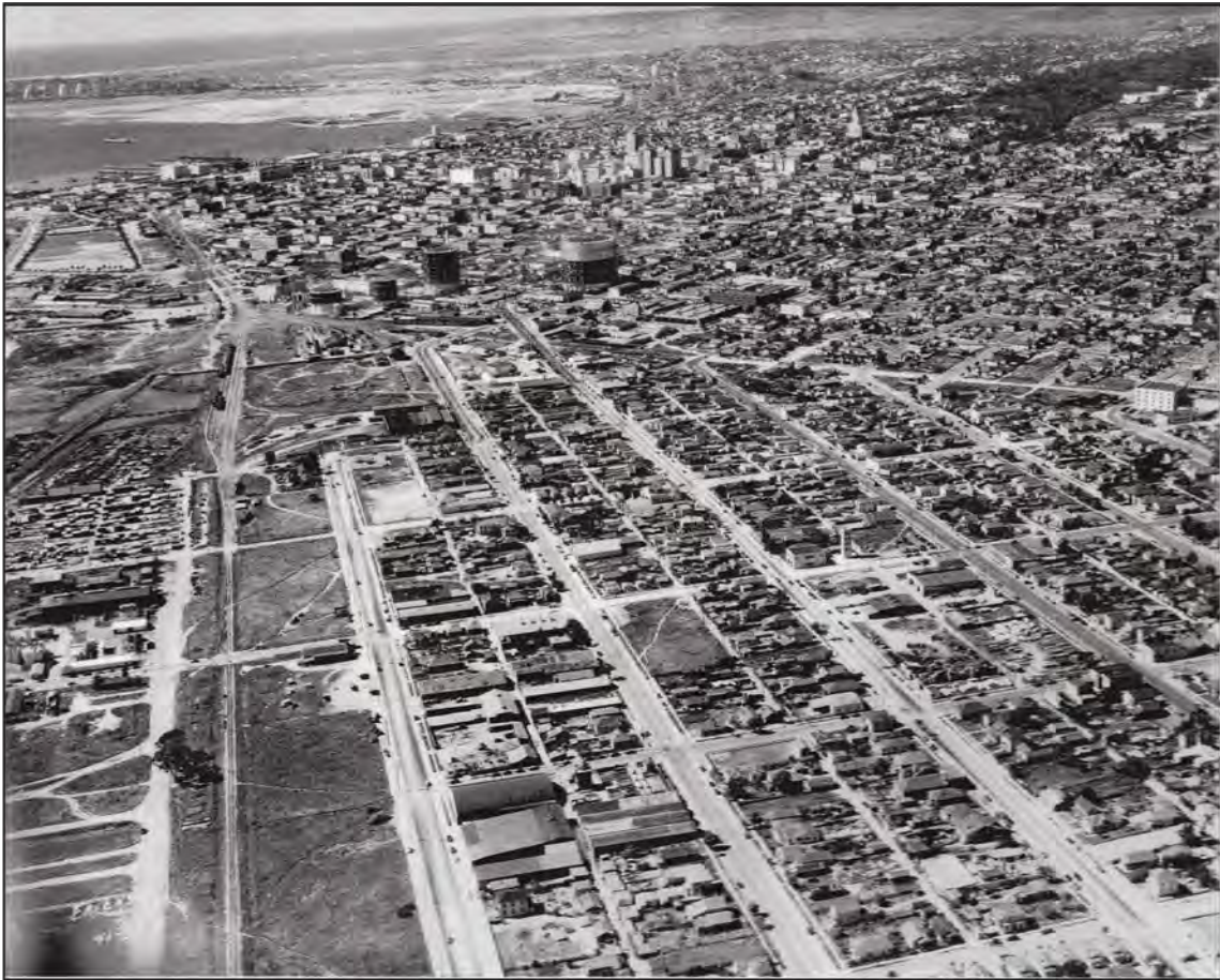
Plate 12. Close-up aerial photograph of the plan area during World War II, facing north. The railroad tracks are on the left side of the frame (left of Main Street). The dirt track to the left of the railroad tracks is Harbor Drive. Note the denseness of development at that time. Many of the buildings had outbuildings or second residences behind. Courtesy of SDHS.
