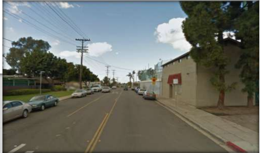
Howard Ave Water Filtration Plant: 2013
