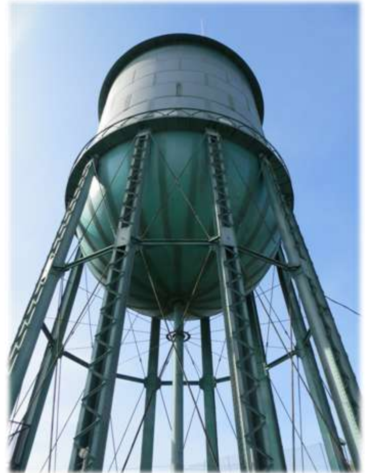
Elevated Water Tank: 2013
