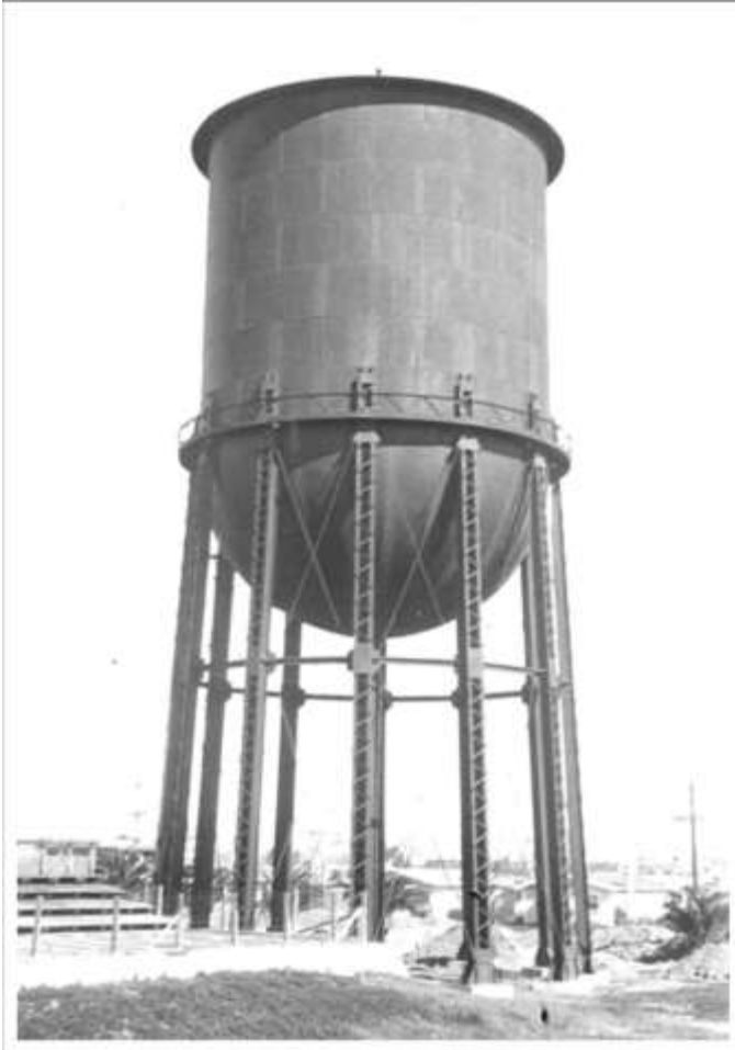
Elevated Water Tank: 1924
