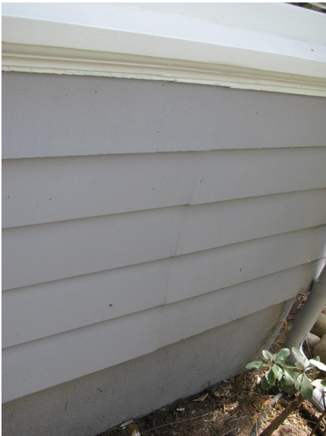
Scarring below right side 1 st story window, June 2013
