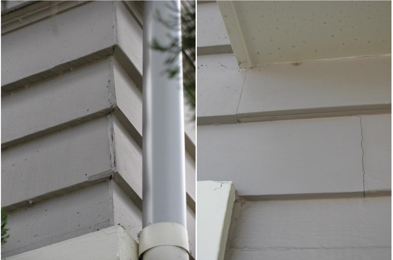
New siding above left side 1 st story window, June 2013
