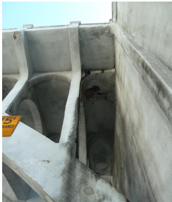
Figure 18. Detail of spandrel arches. Photo taken 2012, IS Architecture.
