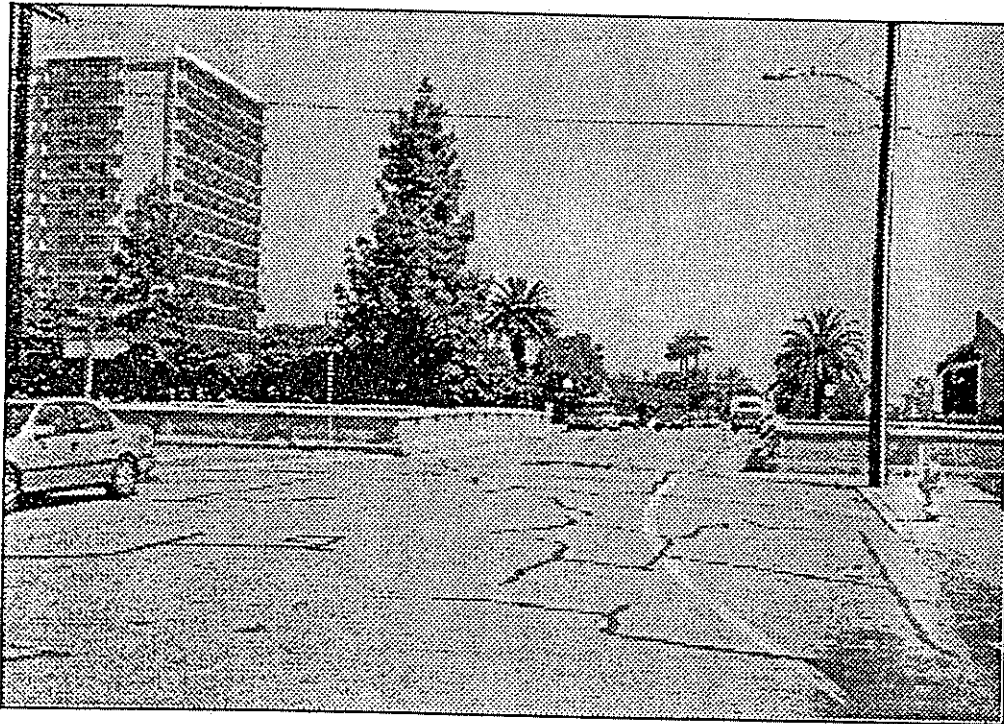
Photograph #3 Georgia Street Bridge/University Avenue Grade Separation Cut Retaining Walls San Diego County, CA Photograph Taken by Alex D. Bevil May 1998 Original Negative in Possession of Photographer View of Southern Approach to Bridge Deck, Looking North along Georgia Street toward University Heights
