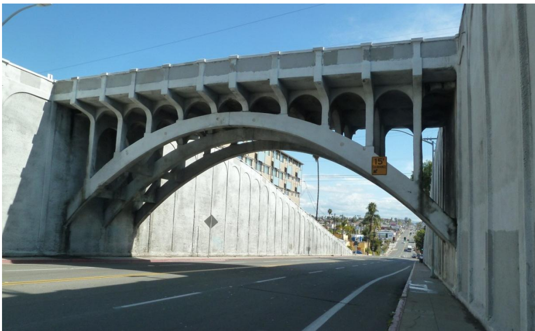
Figure 8. Georgia Street Bridge and grade separation, looking east. Photo taken 2012, IS Architecture.
