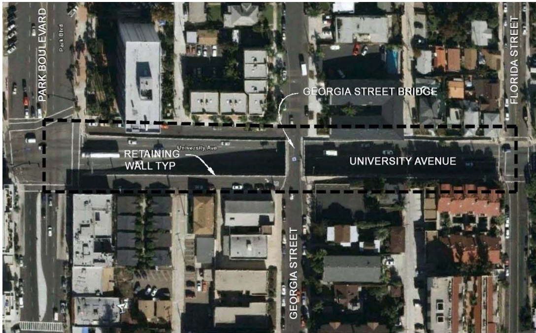
Figure 3. Aerial photograph showing Georgia Street Bridge and grade-separation. Dashed line indicates resource location.
