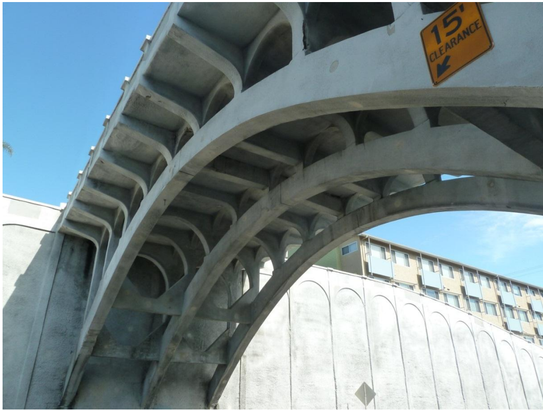
Figure 17. The surface elevation is being proposed to be lowered to meet the vertical clearance required by FHWA.
