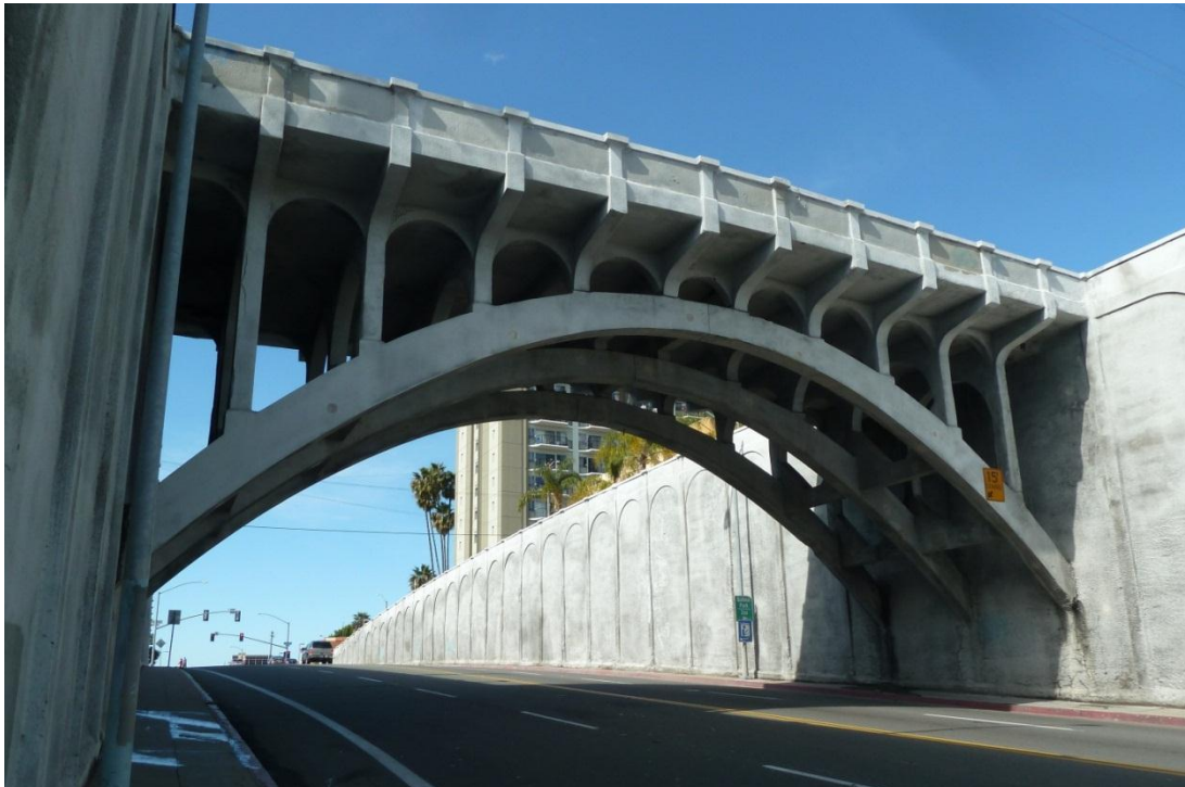
Figure 4. Georgia Street Bridge and grade separation, looking west. Photo taken 2012, IS Architecture.
