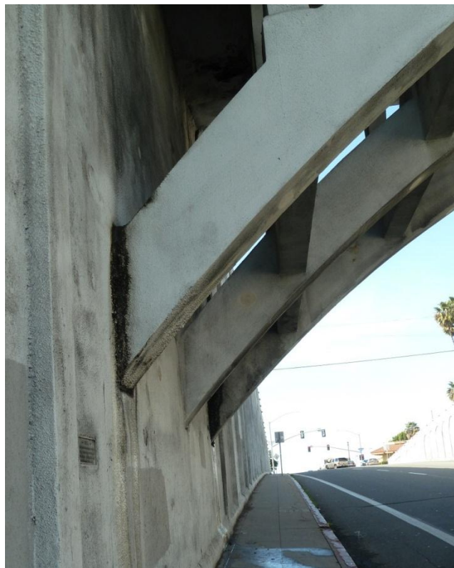
Figure 19. Detail of location of proposed arch end guides. Photo taken 2012, IS Architecture.
