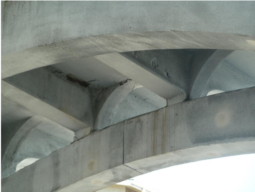
Figure 11. Detail of center arch to be strengthened with the addition of a shear wall. Photo taken 2012, IS Architecture.
