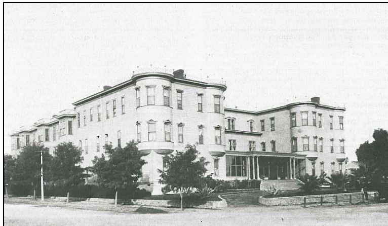
Figure 3. The Florence Hotel, at the corner of Fourth and Fir streets. Source: Elizabeth MacPhail (1979)
