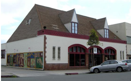
Figure 13: Dixie Lumber & Supply Company building, 2010.
