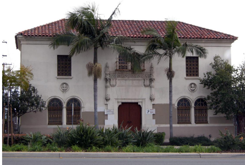
Figure 18: San Diego Gas & Electric Co. Substation F, 2010.
