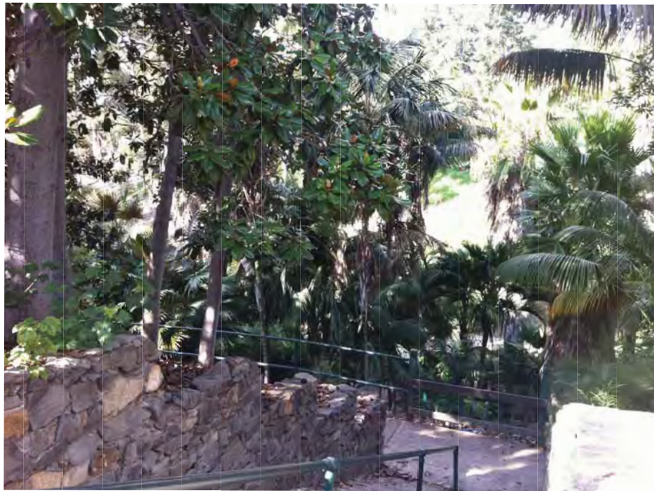
STACKED STONE RETAINING WALL
