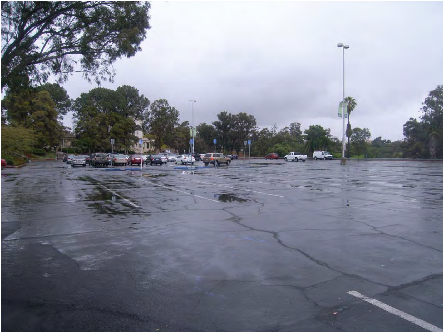
FIGURE 4.3-7 Organ Pavilion Parking Lot
