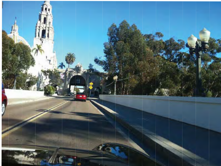
LIGHT SAND FINISH/STUCCO RETAINING WALL
