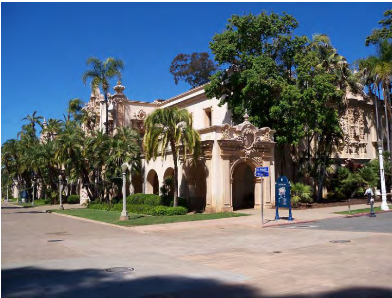
Figure 47. Casa del Prado, view toward northwest Source: Christopher VerPlanck
