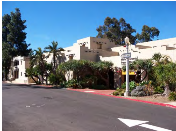
Figure 62. Palisades Building Source: Christopher VerPlanck
