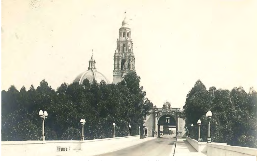
Figure 73. Undated view east on Cabrillo Bridge, ca. 1925 Source: Collection of David Marshall, AIA
