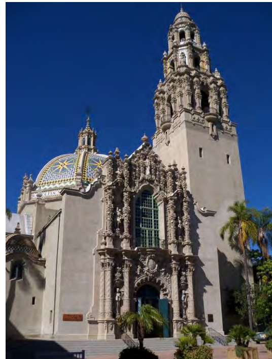
Figure 34. California Building Source: Christopher VerPlanck
