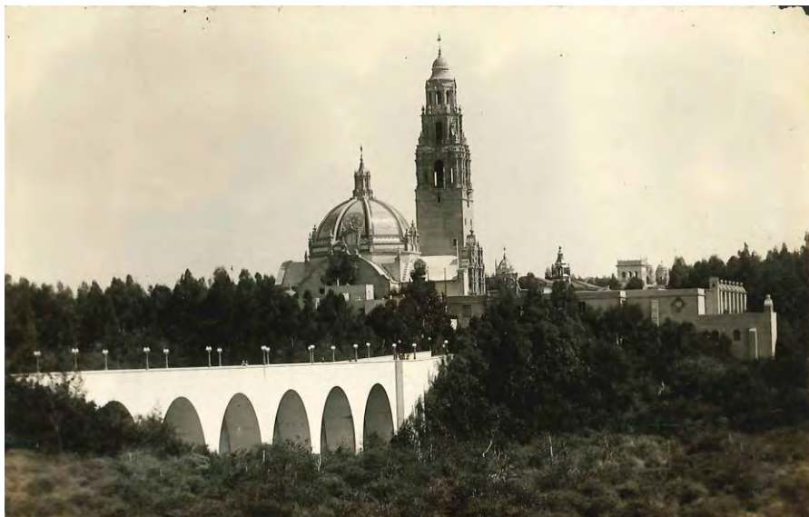
Figure 74. Undated view from West Mesa, ca. 1925 Source: Collection of David Marshall, AIA
