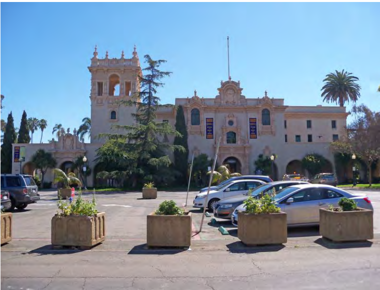
Figure 45. House of Hospitality, looking east Source: Christopher VerPlanck
