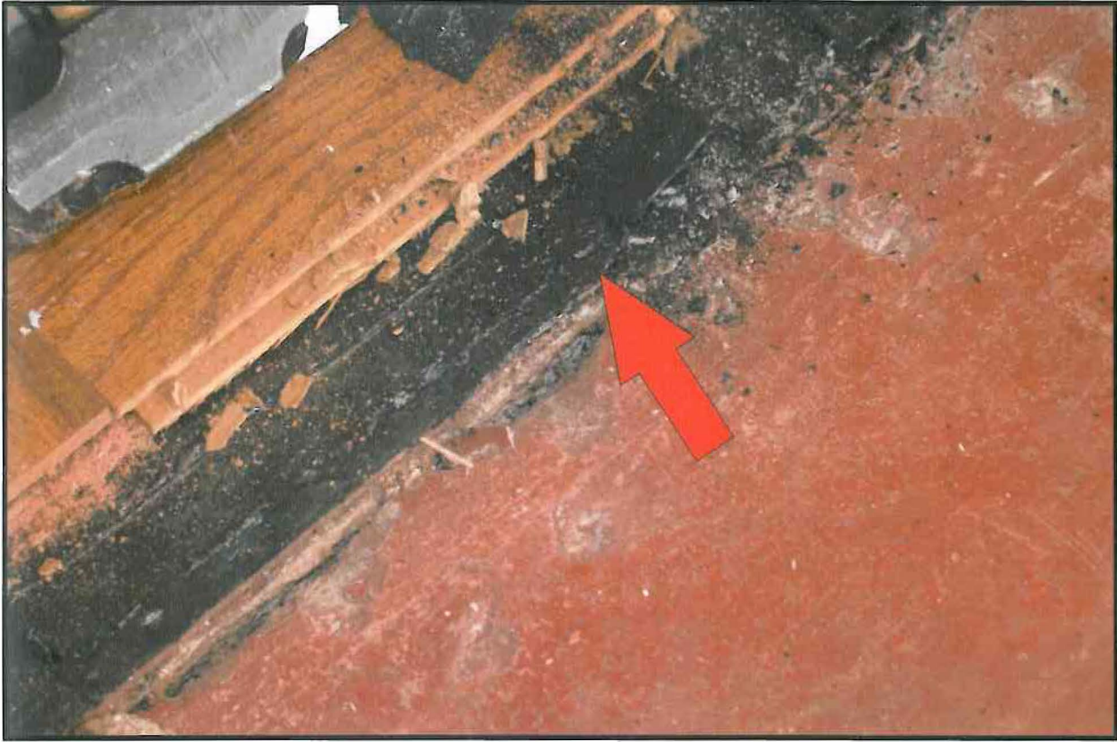
Photo G - Photo of threshold between Living Room and patio showing asphalt sealer to former exterior door.
