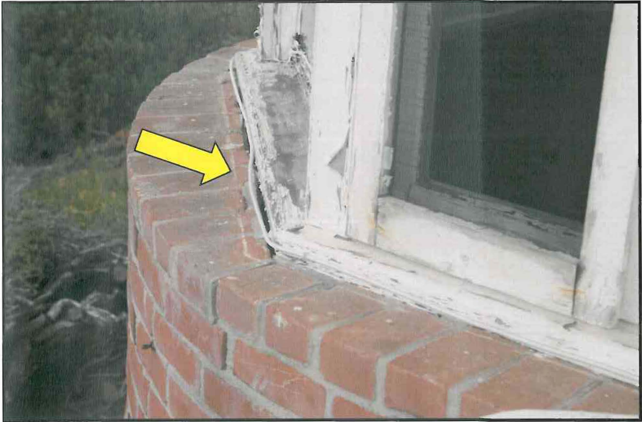
Photo A - Photo showing replaced brick at Kitchen area at rear facade.
