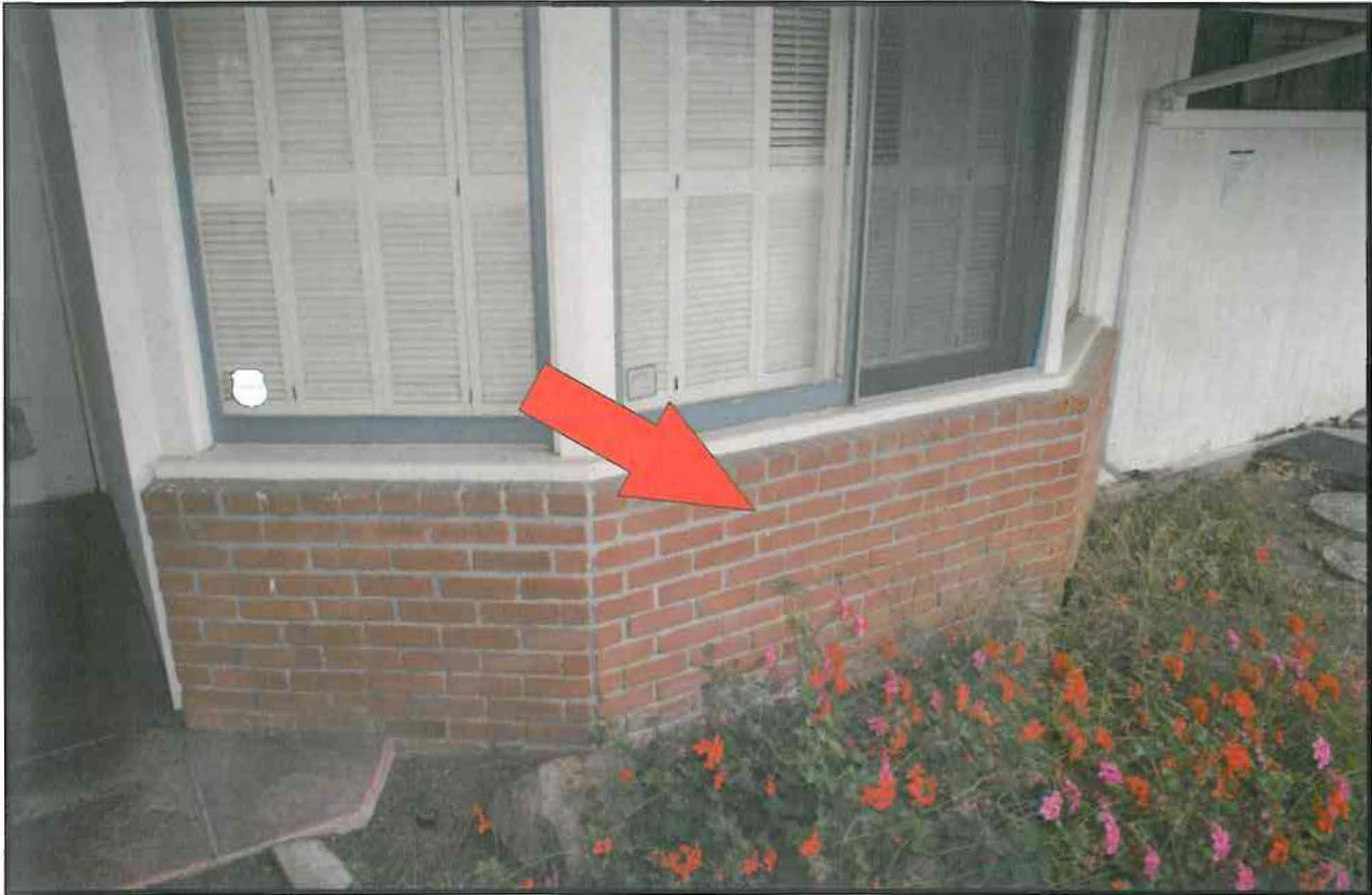
Photo C - Brick cladding at bay window on front facade
