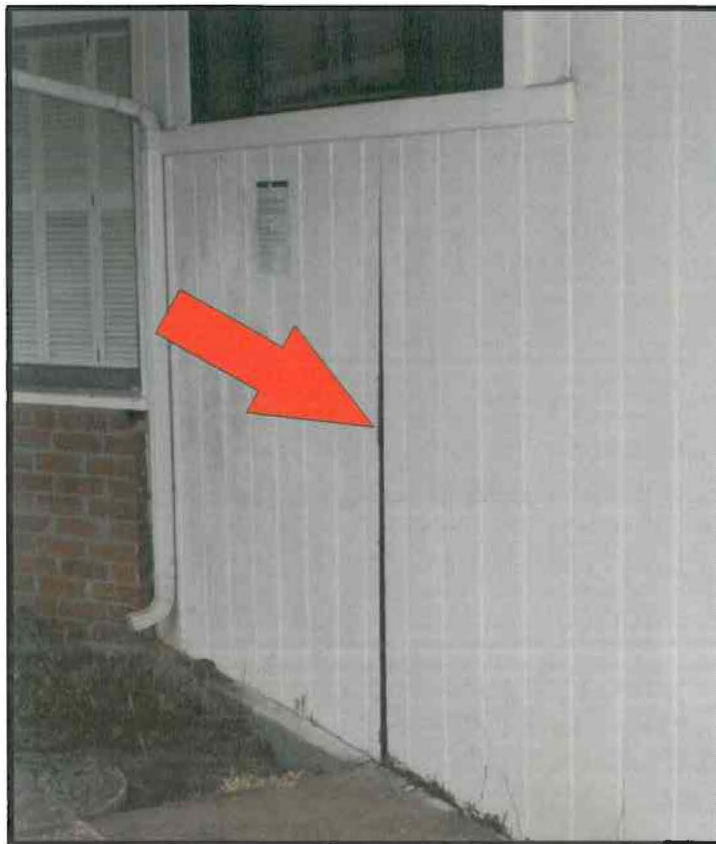
Photo F - Photo clearly showing splice joint in siding under replace window above new foundation
