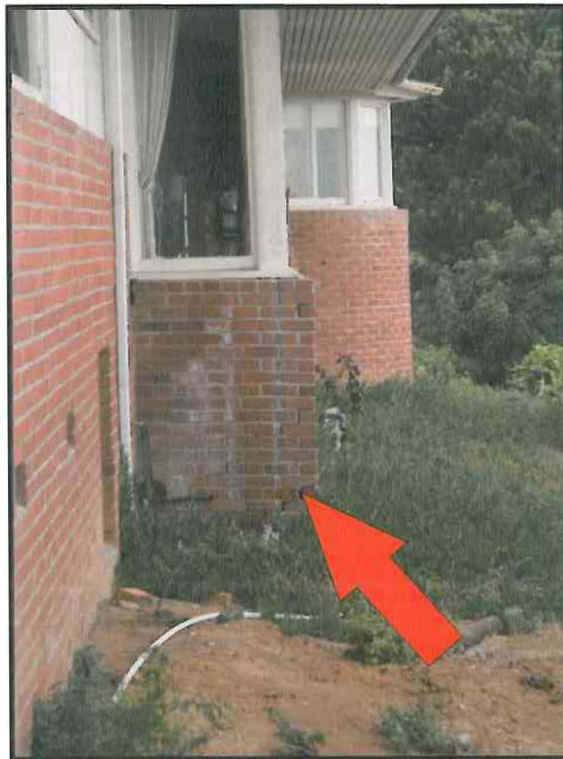
Photo B - Photo showing replaced brick at rear facade.
