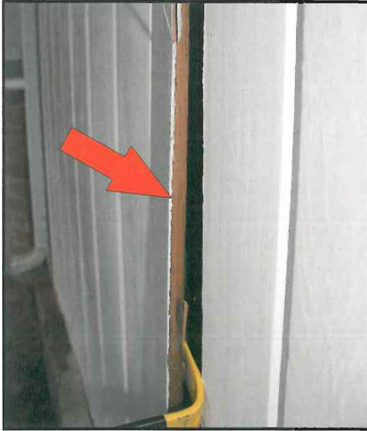
Photo E - Photo showing 45 degree mitre joint mid span on vertical T&G for replaced area of siding under window
