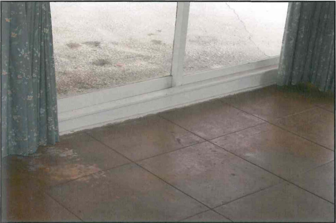
Photo C - Photo showing original scored and colored concrete patio now enclosed - note slope of floor.
