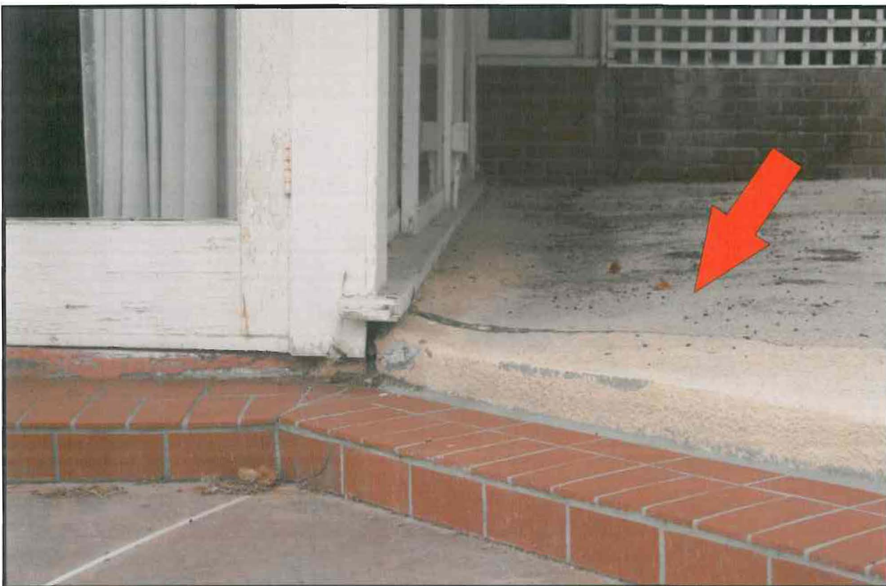
Photo B - Photo showing new concrete patio and finish installed to keep water from flooding home.
