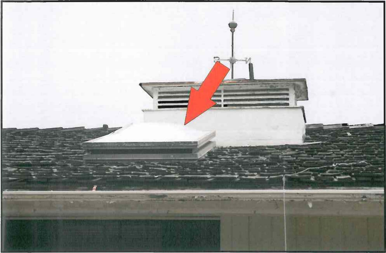
Photo A - Photo showing 4 foot square plastic dome skylight installed at front facade over bathroom.
