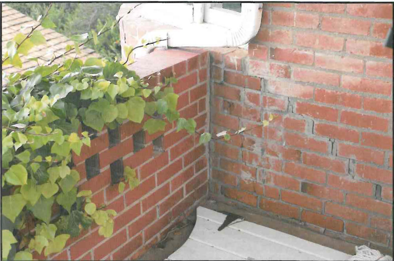
Photo D - Photo showing mis-matched brick at new site retaining walls to house.
