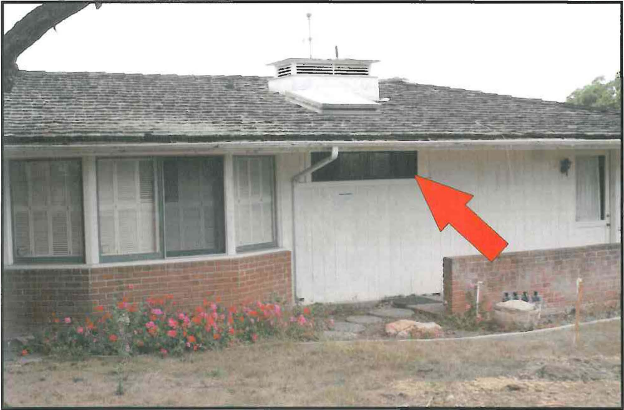
Photo A - Photo showing location of front facade window replaced with aluminum window.
