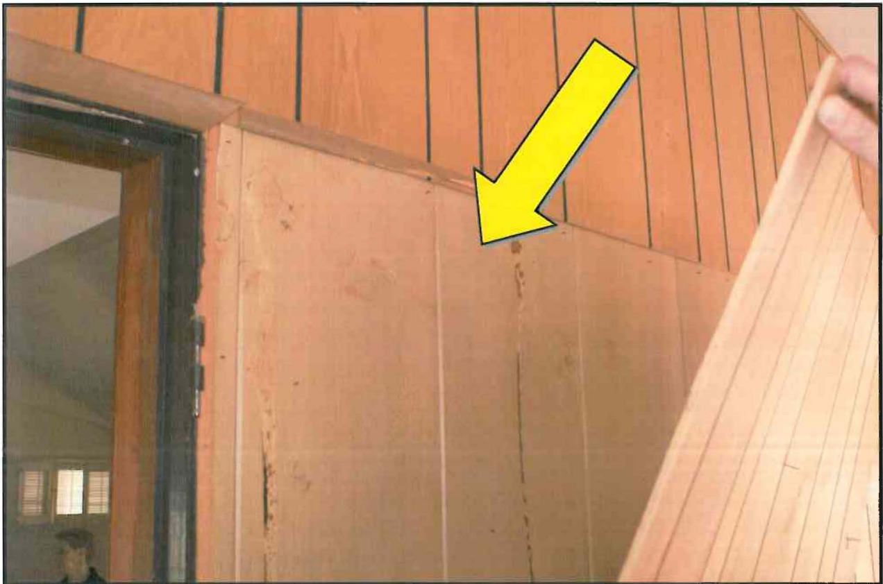
Photo H - Photo showing exterior vertical T & G siding behind paneling in former patio room .
