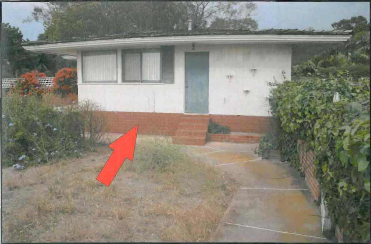
Photo A - Photo showing applied non-original "brick" veneer to garage
