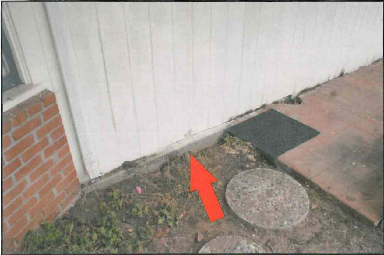
Photo C - Photo showing area of new foundation under replaced window (see color of concrete).
