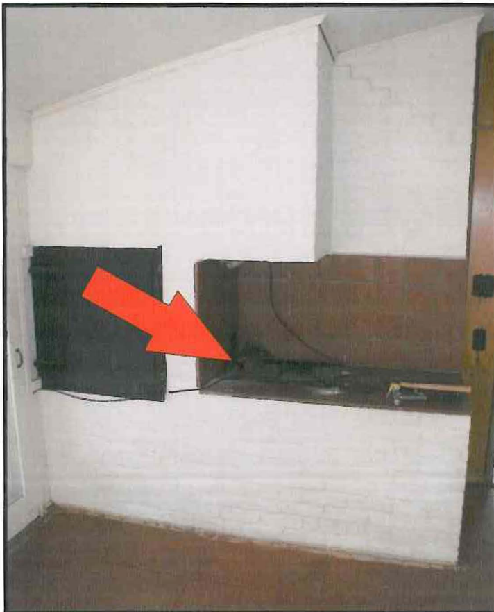
Photo F - Photo showing exterior barbeque located at now enclosed patio without full exhaust covering even.
