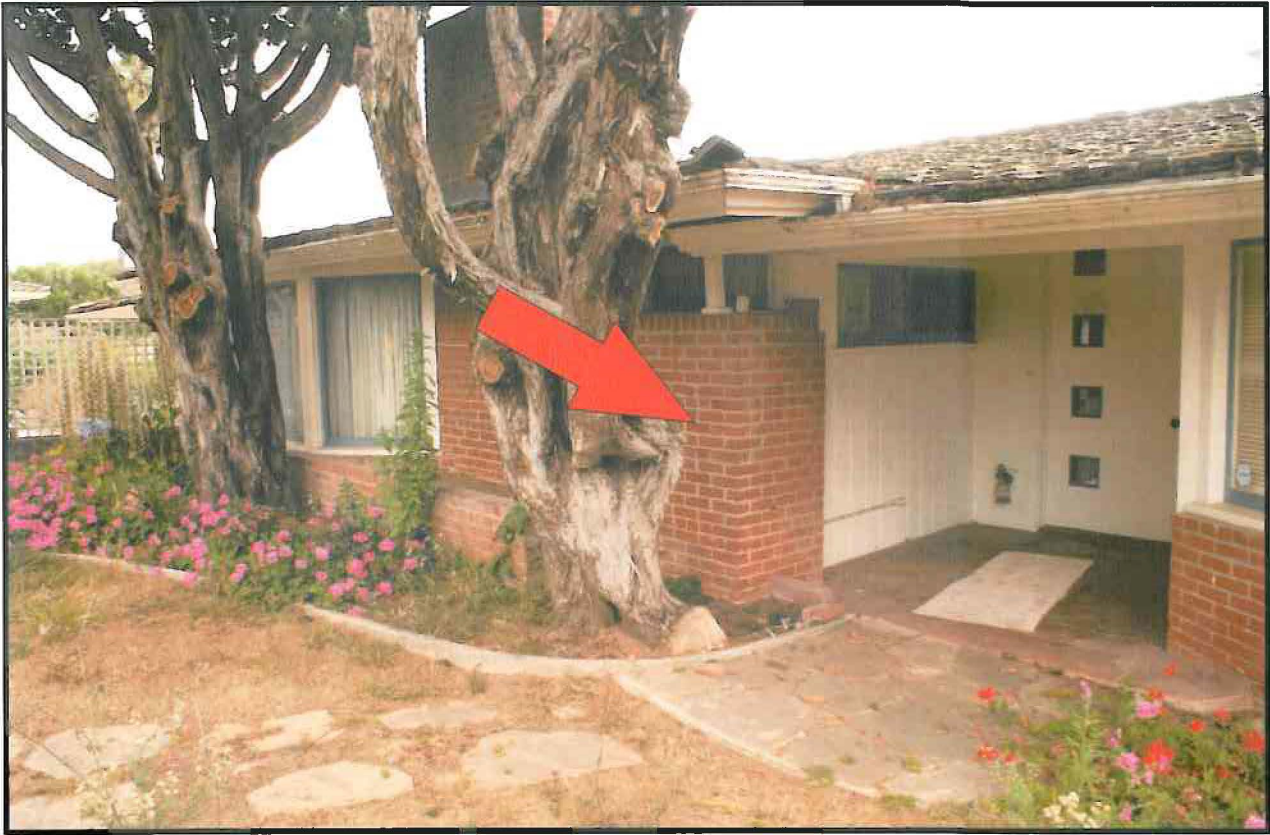
Photo A - Photo showing brick area adjacent to fireplace
