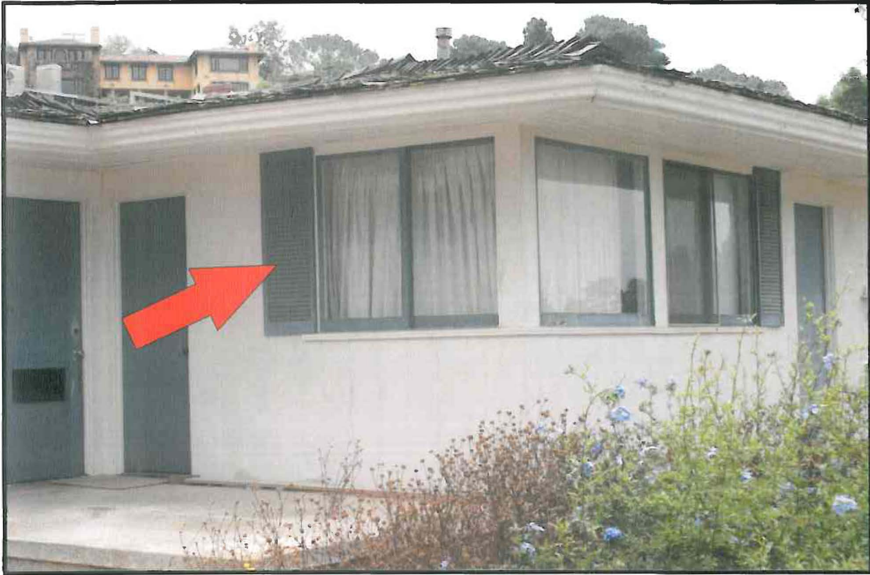
Photo A - Photo showing the only 2 shutters on the home which are not true shutters but tacky ornament.
