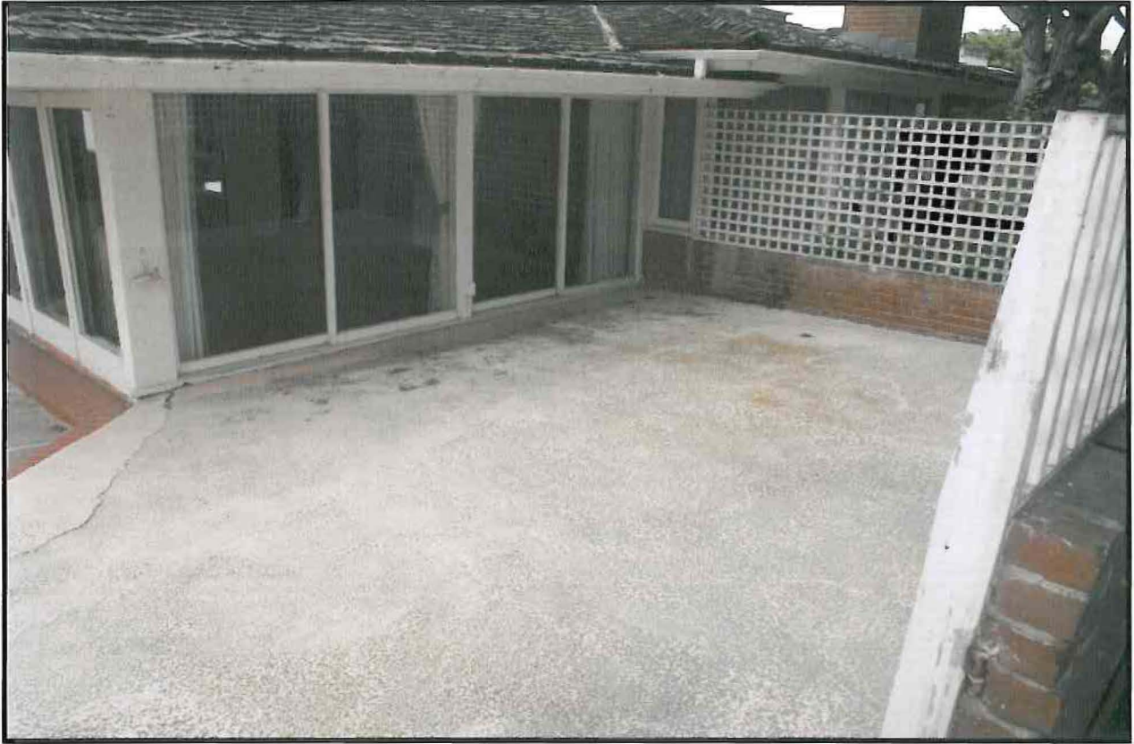
Photo A - Photo showing enclosed patio area at front southern corner of the home.
