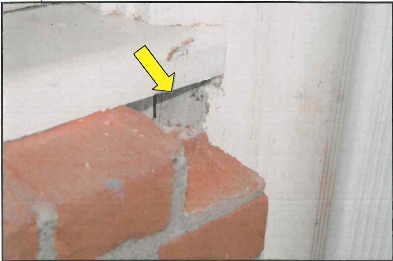
Photo D - Photo showing wood siding installed behind brick cladding
