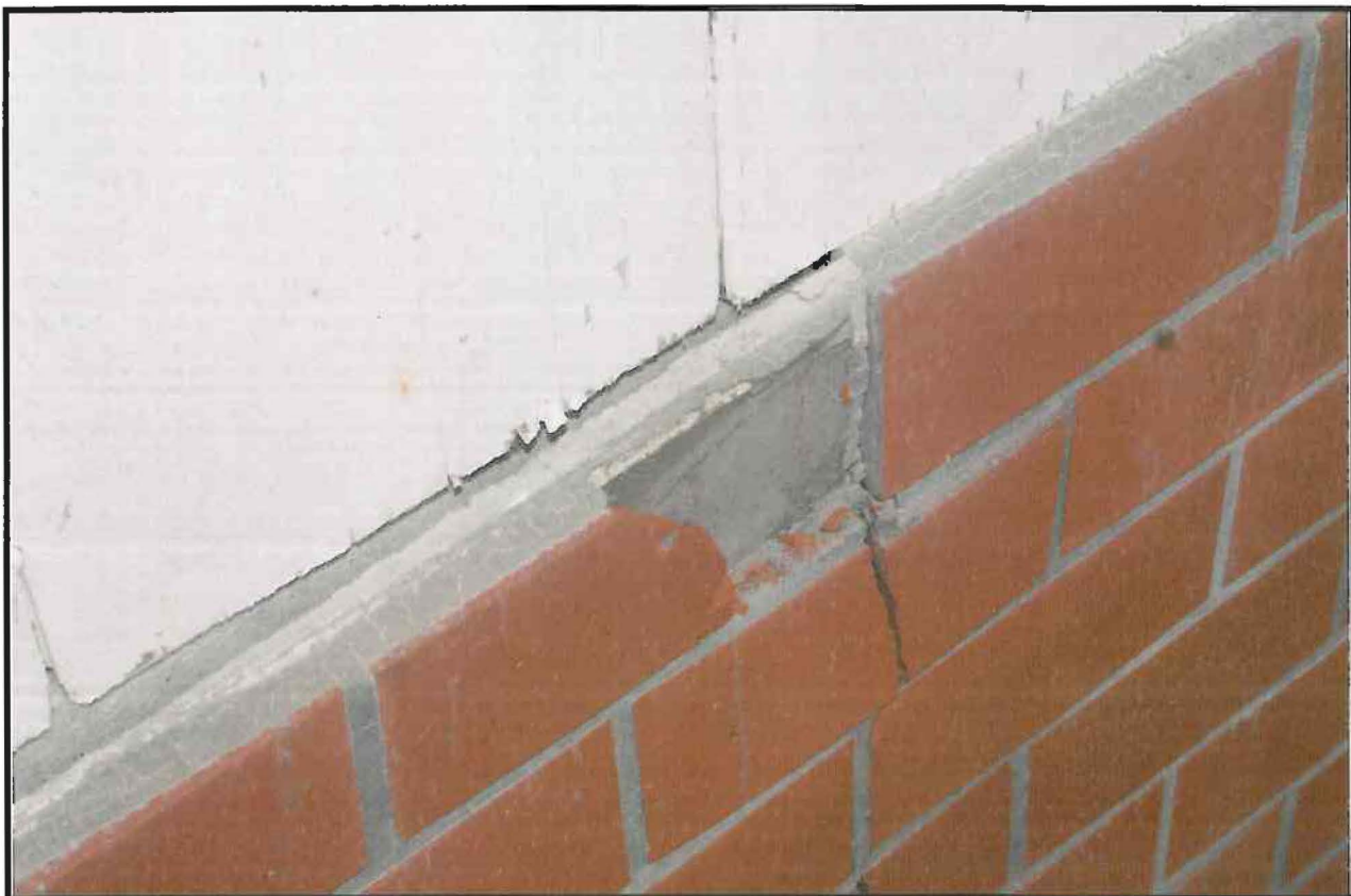
Photo B - Photo showing applied non-original "brick" veneer to garage.
