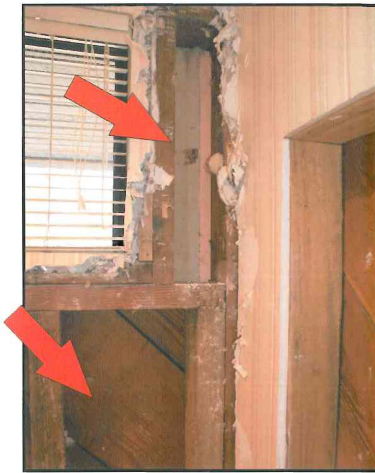
Photo I - Photo clearly showing re-framing of side and bottom at replaced window and new skip sheathing
