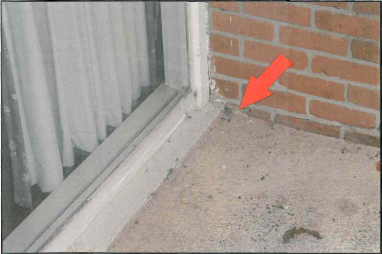
Photo C - Photo showing new concrete patio poured to top of added wood window sill.
