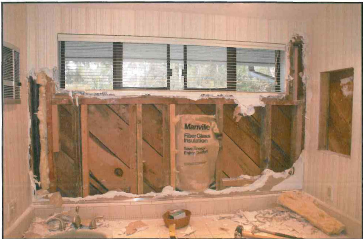
Photo H - Photo clearly showing complete re-framing at replaced window
