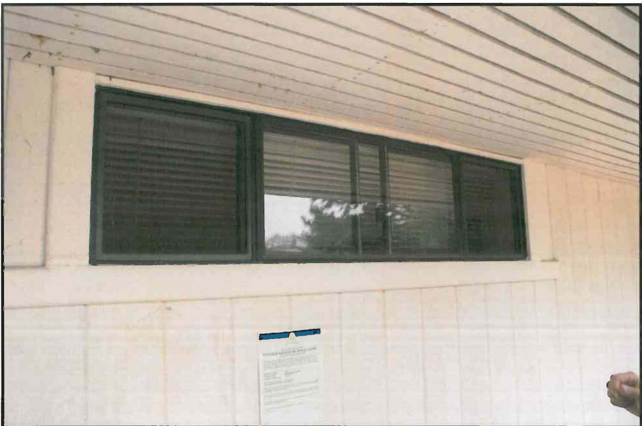
Photo B - Close up showing aluminum replacement window.
