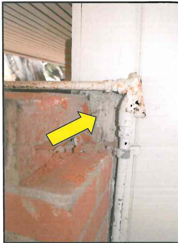
Photo B - Photo of brick at entry area showing wood siding behind the brick .
