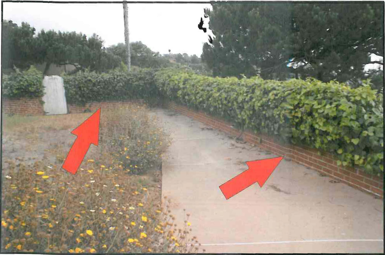
Photo A - Photo of new site walls and retaining walls added .
