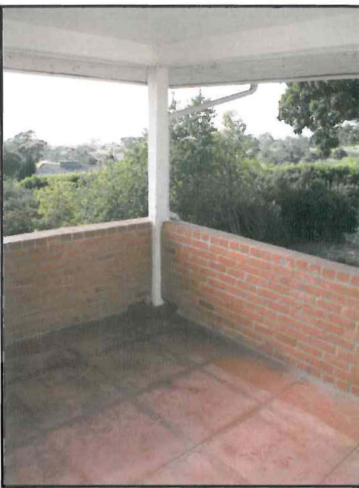
Photo E - Reference photo showing exactly the same scored red concrete at northwestern open patio.
