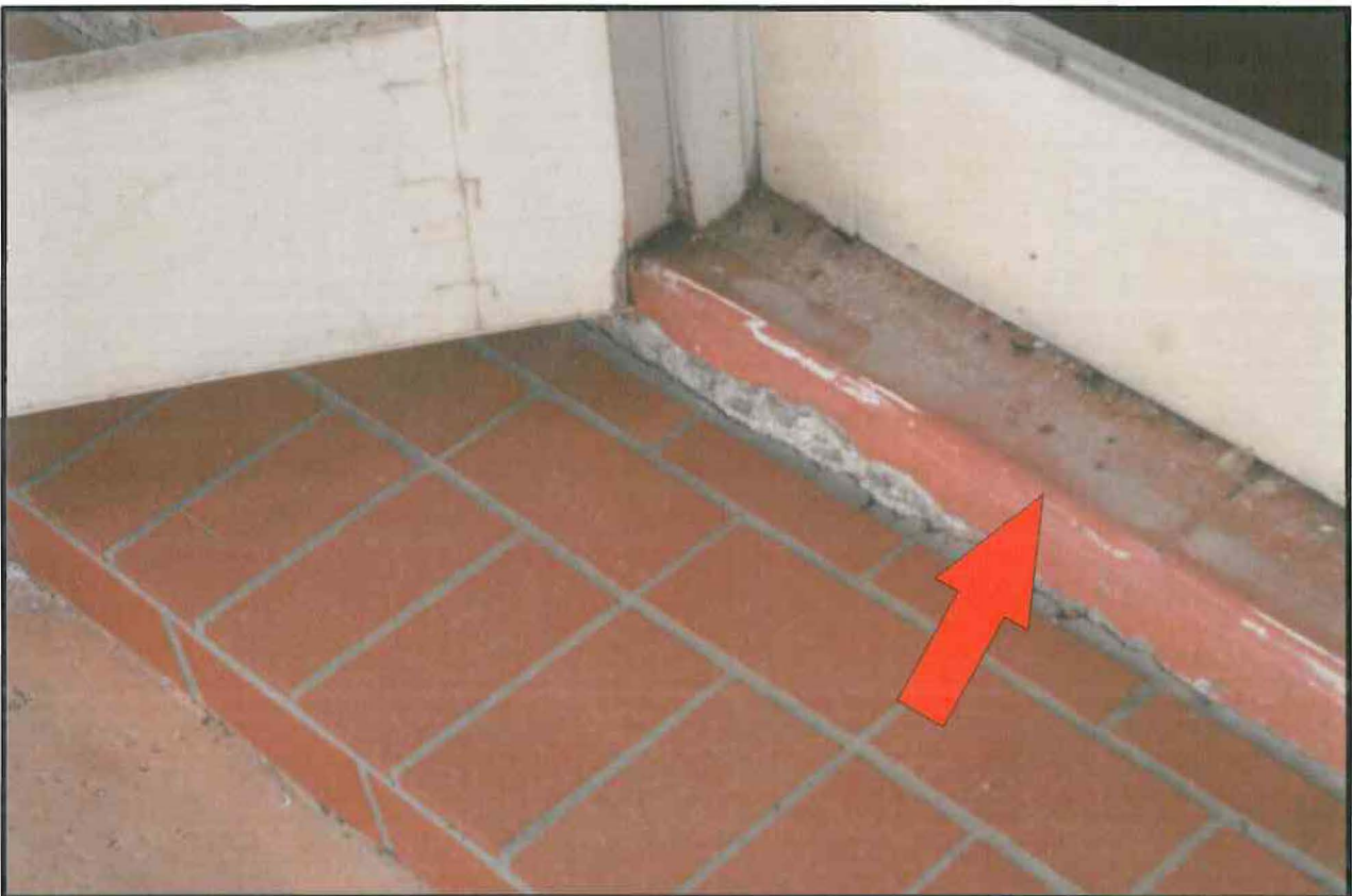
Photo D ~ Photo showing original patio edge in red concrete with wood doors place on top.
