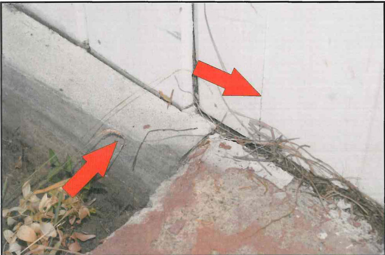
Photo D - Photo showing clear evidence of new foundation and vertical joint in T&G siding.
