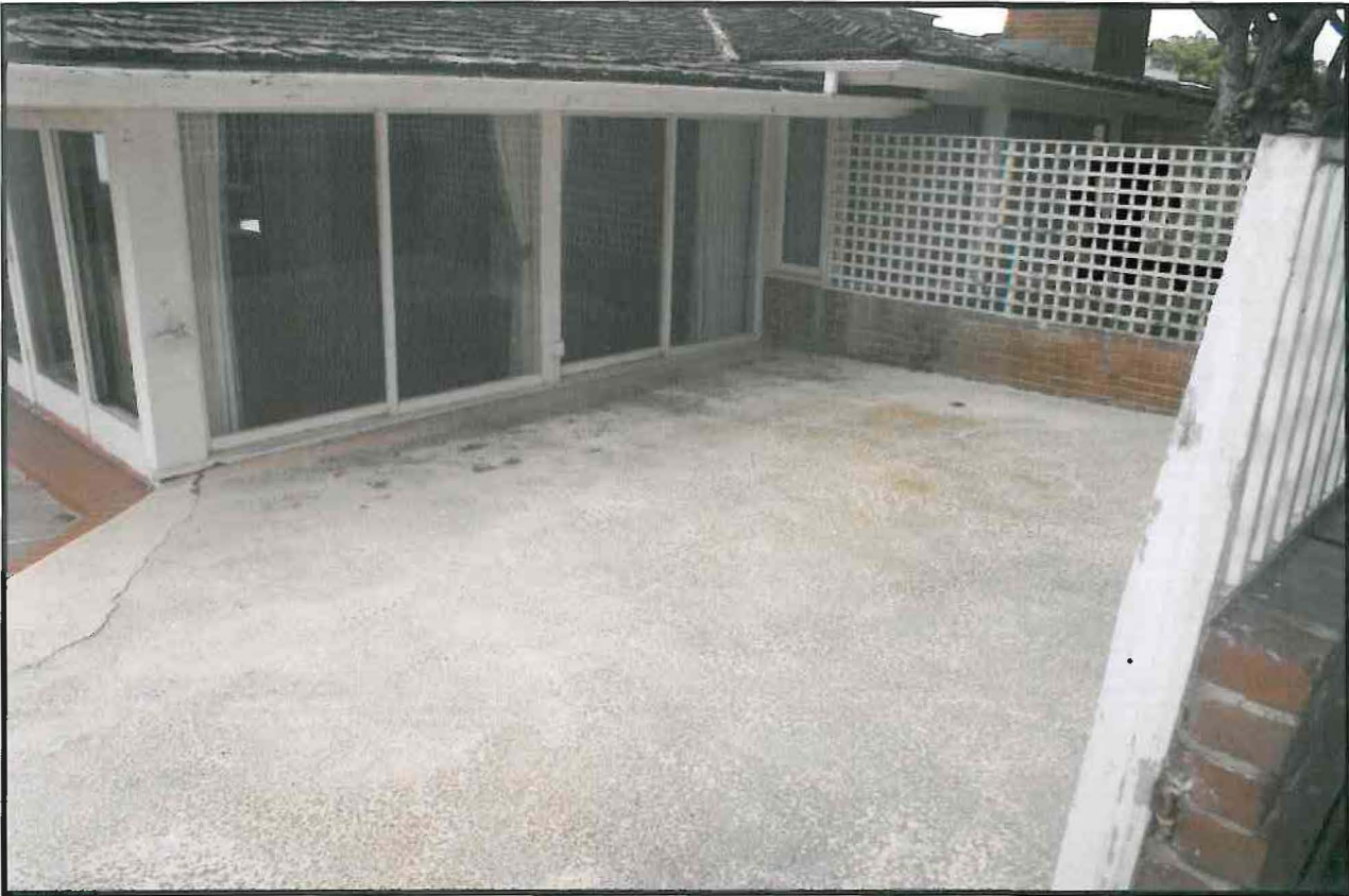
Photo A - Photo showing new concrete patio and finish installed to keep water from flooding home.
