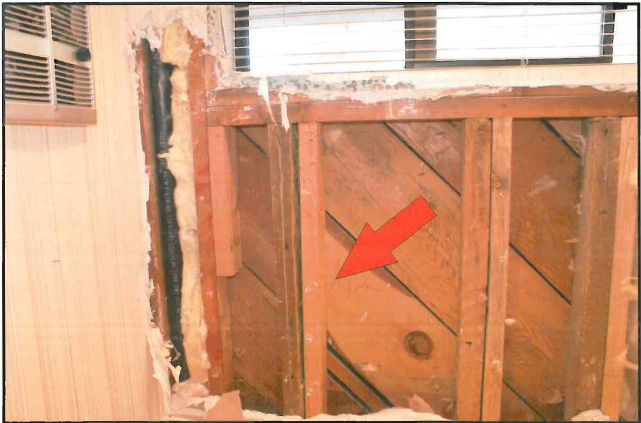
Photo J - Photo clearly showing re-framing of side and bottom at replaced window and new skip sheathing
