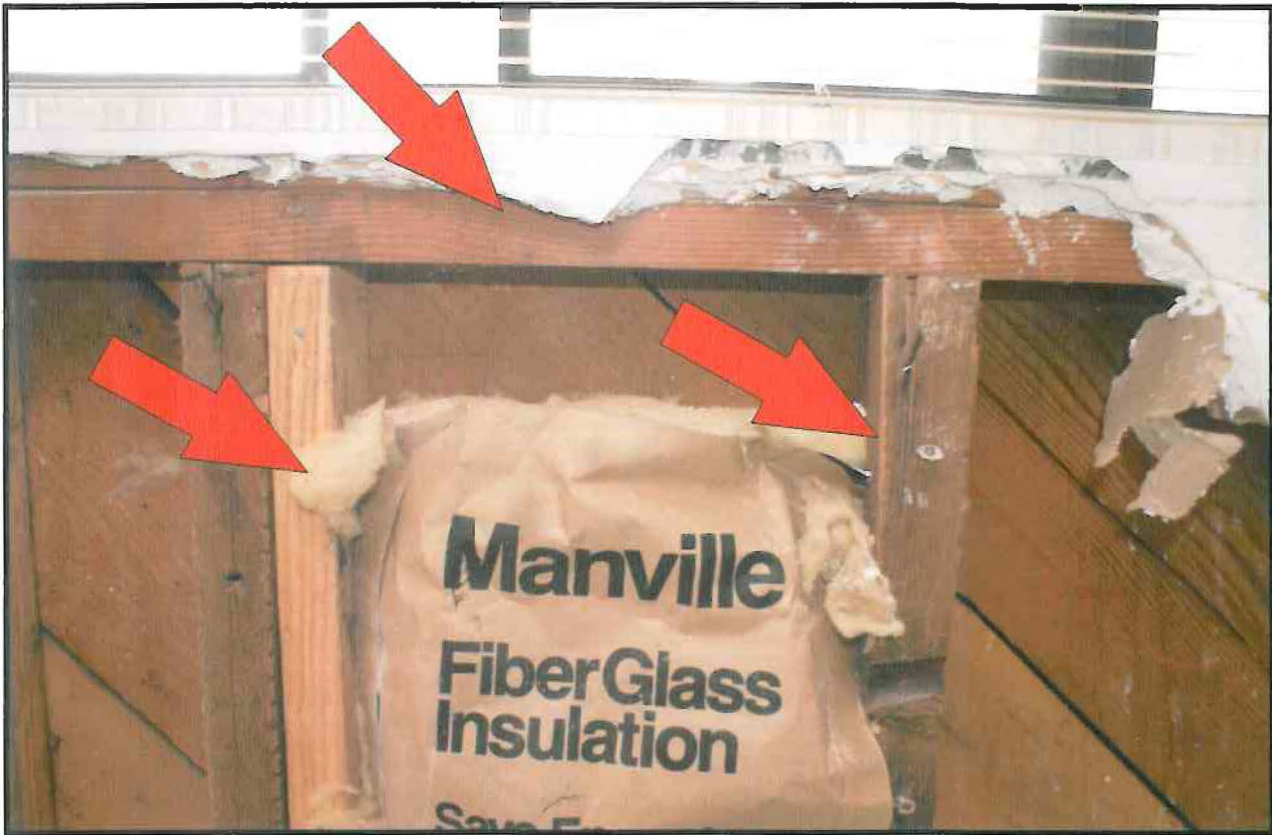
Photo G - Photo clearly showing at least 3 generations of framing lumber at replaced window
