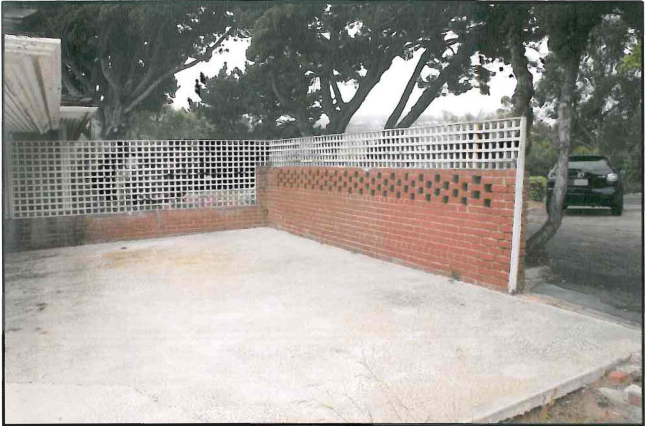
Photo A - Photo showing added and remodeled brick site wall visible to front elevation
