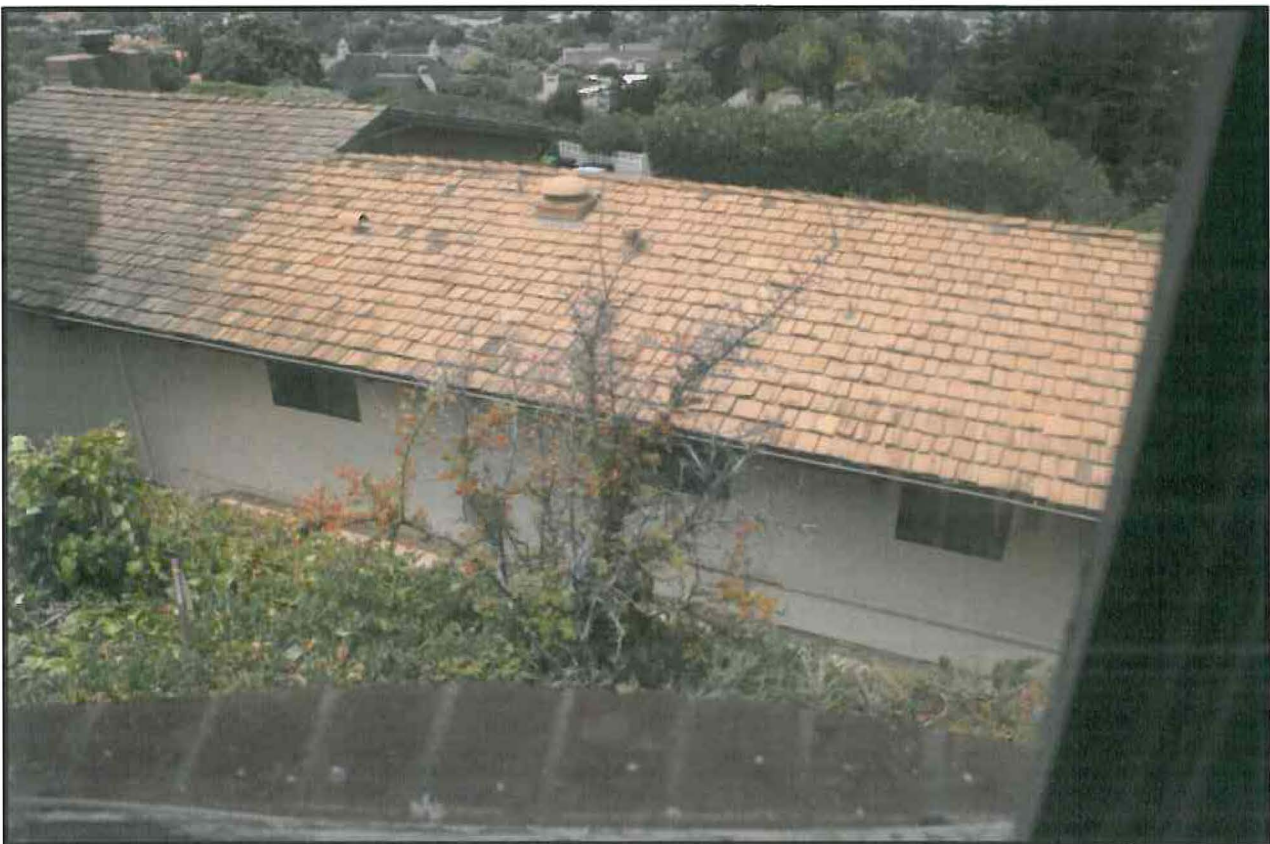
Photo D - Photo from 6604 Residence Kitchen showing proximity of post-lot split adjoining home.
