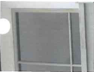
Hopper Windows Replaced with Fixed Panes
