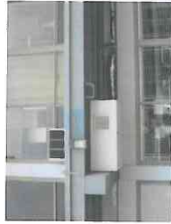
Awning Transom Replaced with Venting Door
