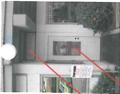
Glazing Removed From Awning Transom Over Door
