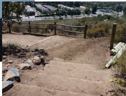
Photos from Cowles Mountain Trail Repair work
