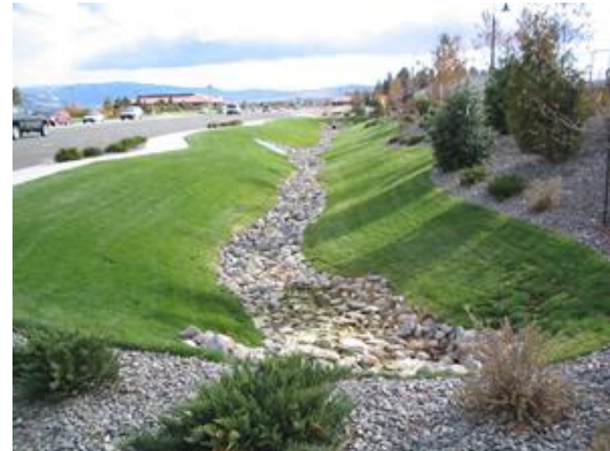
Example of a swale
