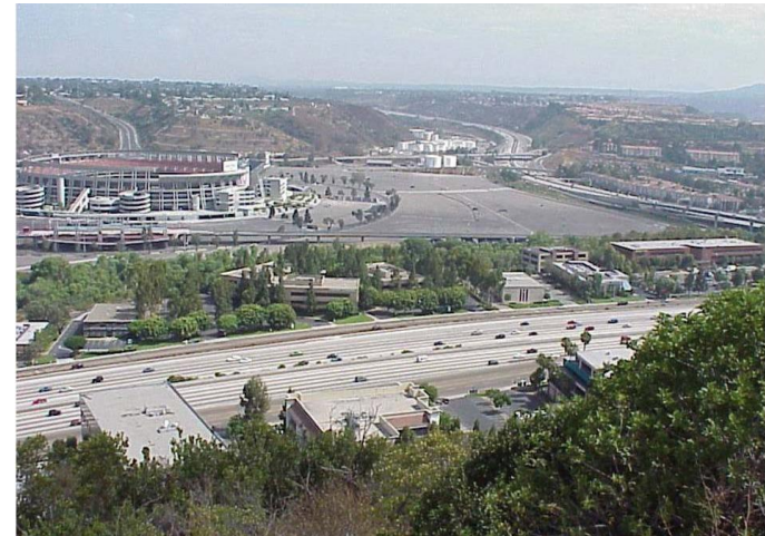
Qualcomm Stadium Site
