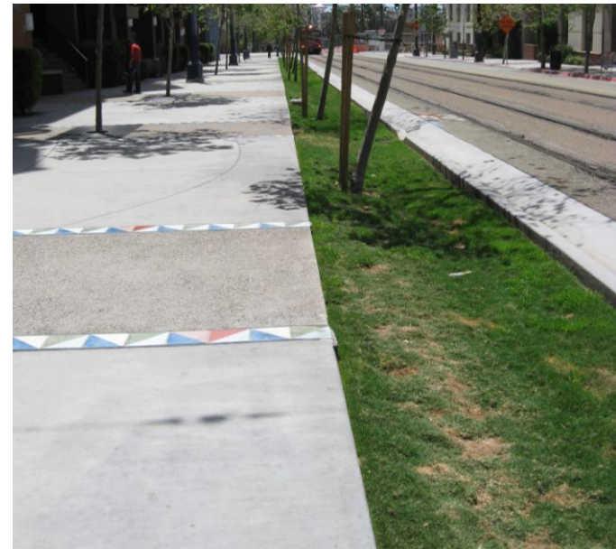
Example of an infiltration basin
