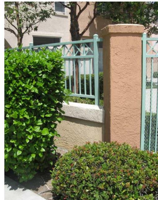
3' wall, with 3' high, 75% transparent fence attached
