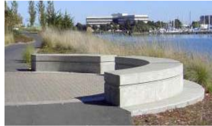
Concrete seat walls located adjacent to multi-use path
