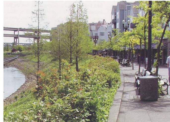
Example of manufactured slope and native planting between path and river at approximately 3:1 slope
