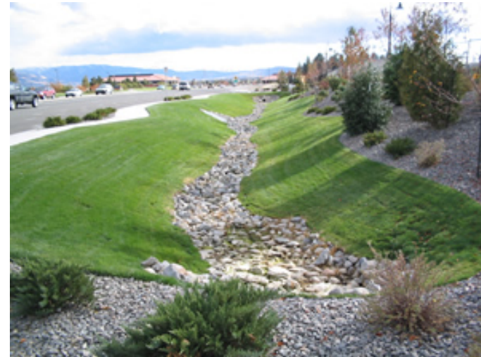
Example of a swale
