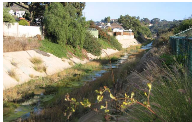
Hard surfaced channels such as Tecolote Creek increase velocity, prevent groundwater recharge and offer little wildlife habitat
