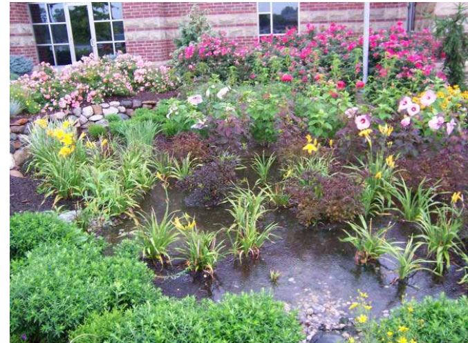
Example of an infiltration basin
