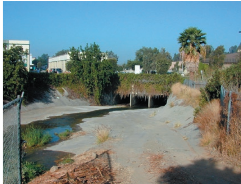
Channelized Alvarado Creek above Grantville Post Office
