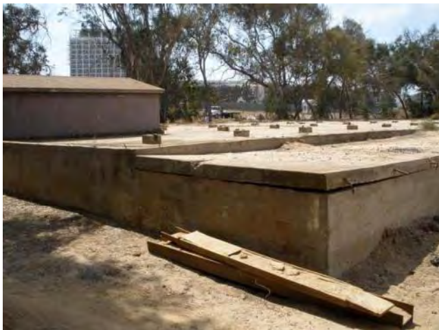
Camp Callan Post Office foundation, on UCSD property
