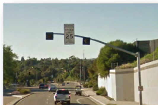
Advance school signage – not compliant with 2010 MUTCD
