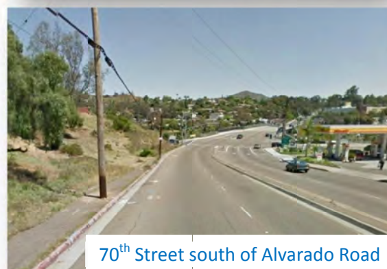
West side of 70 th Street
