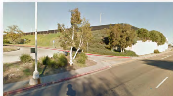
Obstructed sidewalk and lack of proper curb ramps
