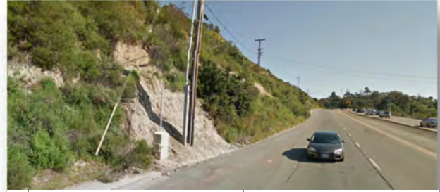
Northbound Fairmount Avenue – discontinuous sidewalk north of Aldine Drive on-ramp
