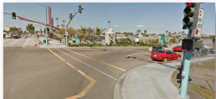
Entrance to I-15 NB on-ramp – at Central Avenue
