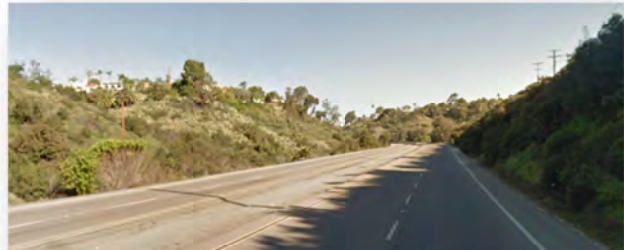
Fairmount Avenue – no sidewalks on either side (grade issues?)
