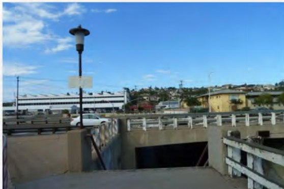
Entrance to pedestrian underpass on south side of Pacific Highway
