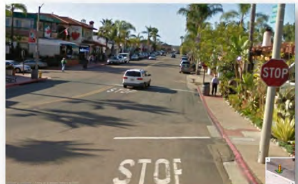
Five-legged intersection difficult to navigate at Linwood Street / Conde Street
