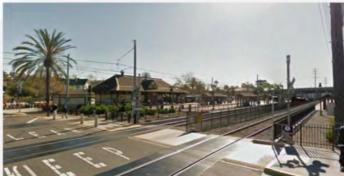
No signage or pedestrian crossing signals at train tracks on Taylor Street
