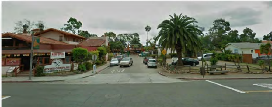
Missing concrete sidewalk at Congress Street / Twiggs Street
