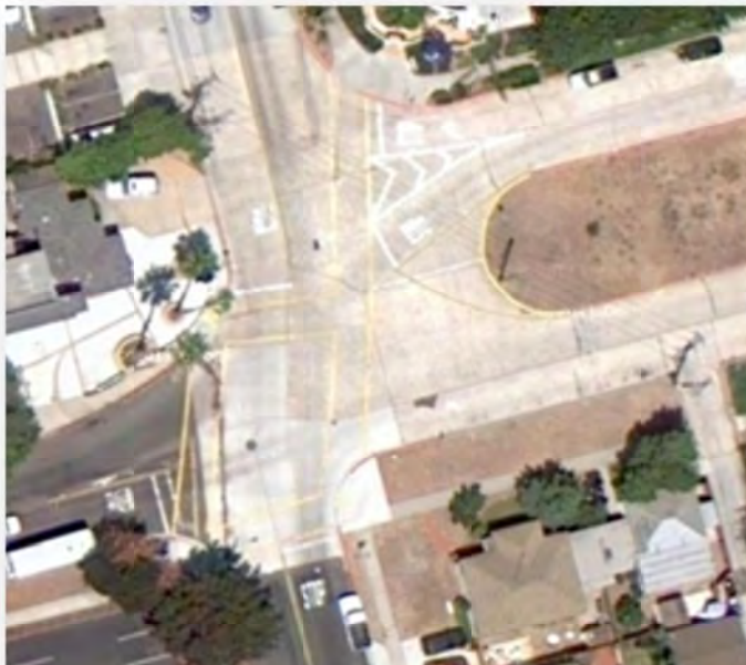
Couplet on Pacific Beach Drive creates long skewed crossing distances
