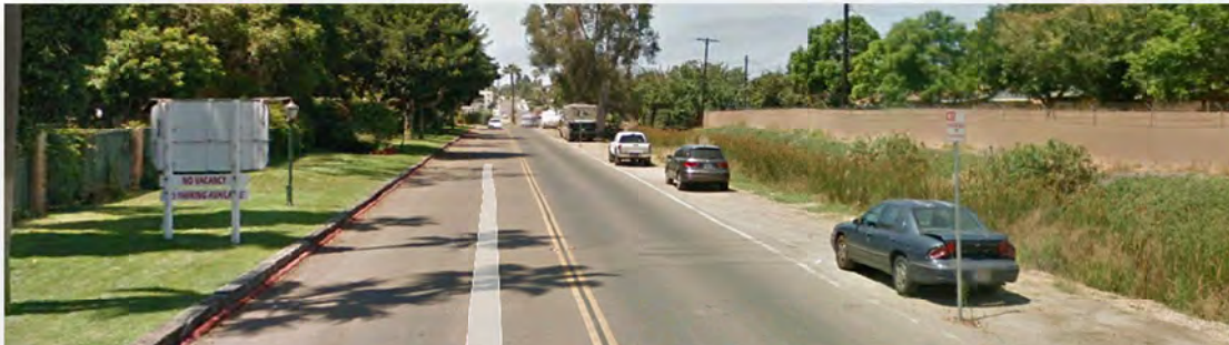
Missing sidewalks on Pacific Beach Drive
