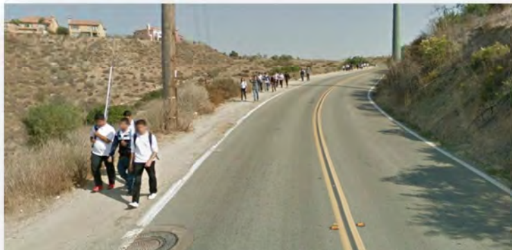
Children walking in street due to missing sidewalk
