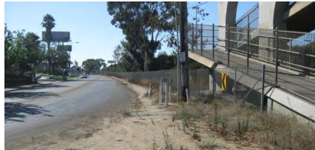
Insufficient lighting near pedestrian bridge
