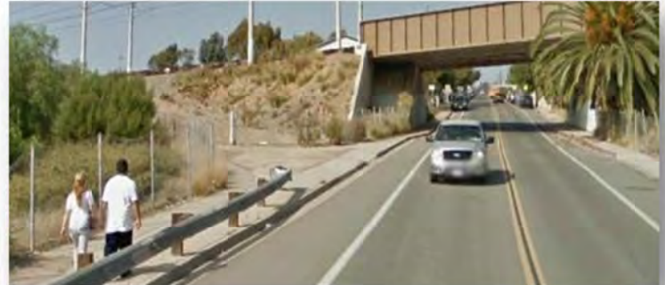
Access from E. Beyer Boulevard to pedestrian bridge crossing I-805
