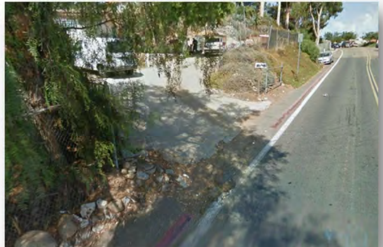
Asphalt shoulder along North Lane
