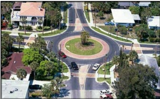
18S) Roundabout. Photo credit: Michael Ronkin
