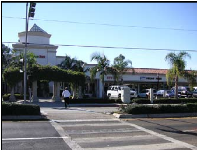
13S) The response time for stopping traffic for this mid-block crossing was quick, assuring that pedestrians will tend to wait for the lights. The design of the adjacent walkways concentrated pedestrians into this walkway crossing. Photo credit: Mike Singleton
