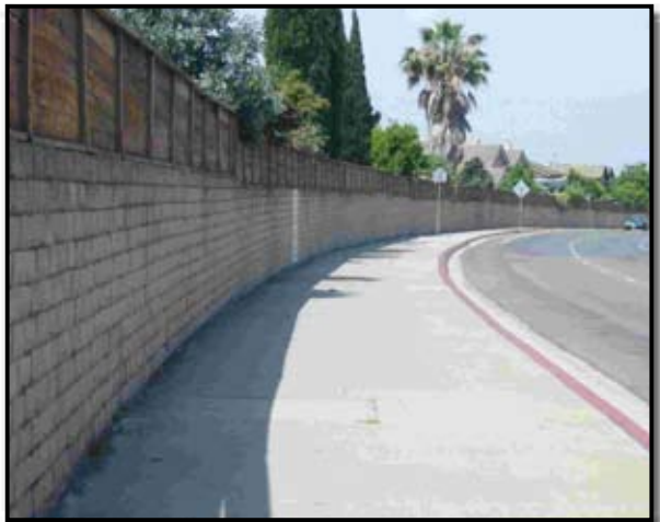
Wide but unbuffered sidewalk (Mira Mesa Boulevard near Parkdale Avenue)
