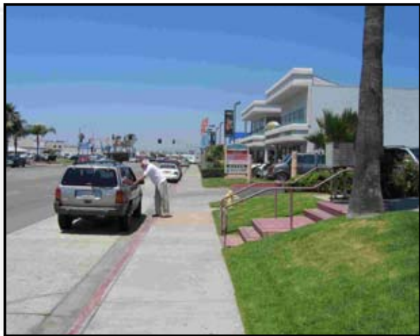
Sidewalk at curb (Convoy Street at Engineer Road)
