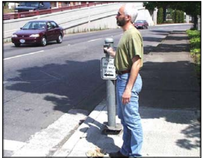
2A) Pole mounted ped. signal actuator placed in accessible area next to the curb ramp. Photo credit: Michael Ronkin
