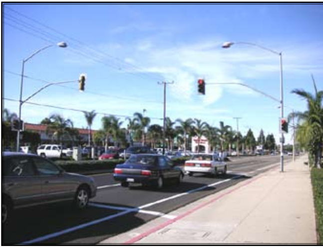
13S) This mid-block crossing utilizes standard traffic signals, a stop bar, ladder style crosswalks, median refuge and a pedestrian controlled actuator. Photo credit: Mike Singleton
