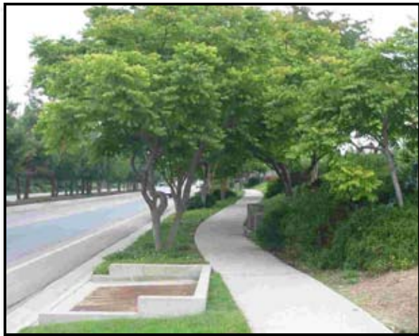
Buffered sidewalk (Scripps Poway Parkway near Spring Canyon Road)
