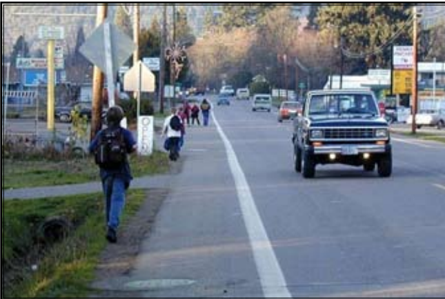
2C) Where signs of continual pedestrian use are present along higher volume and higher speed streets, the addition of sidewalks should be a top priority. Photo credit: Michael Ronkin
