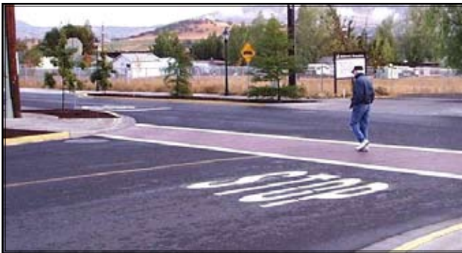
3S) Increased visibility can be obtained through a change of paving materials and striping. Photo credit: Michael Ronkin
