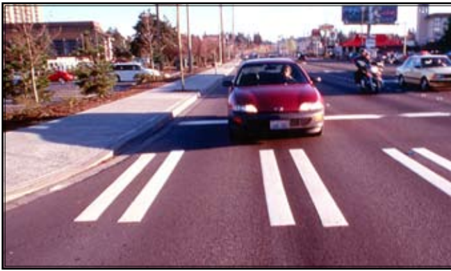
3S) Ladder style markings can be modified and spaced to lower the wear from vehicle tires. Photo credit: Dan Burden
