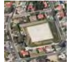
Bayview WPS and Reservoir
