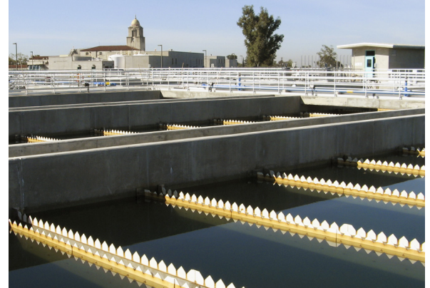
Alvarado Water Treatment Plant
