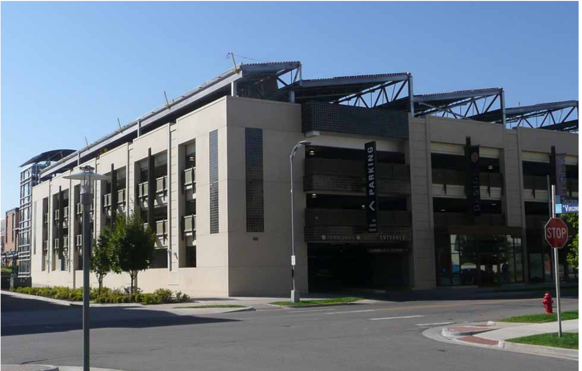
parking garage with solar panels
