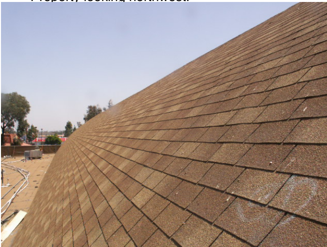
The barrel roof at the skating rink has combination shingles.
