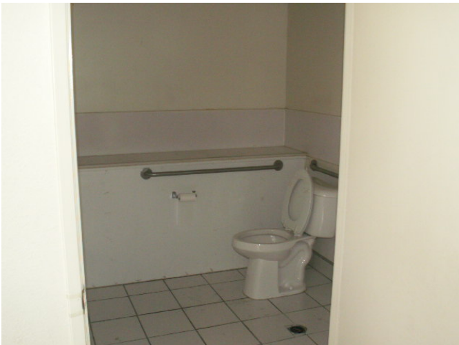
View of the public restroom at the medical office.
