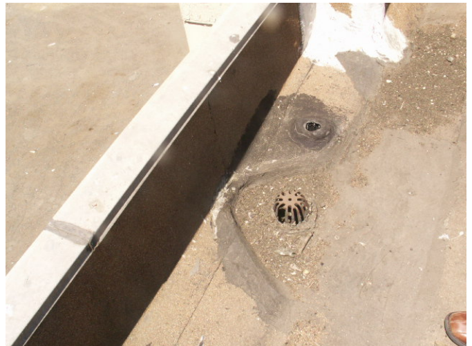
In addition to scuppers and downspouts, there is a roof drain and overflow on the flat portions of the roof.
