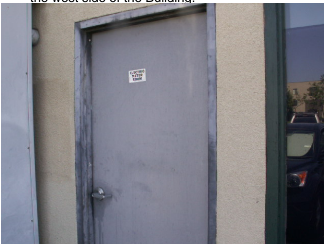
The door to the electrical room requires paint.
