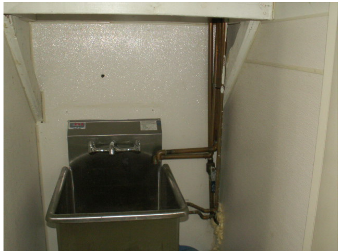
Copper piping is used for the plumbing throughout.
