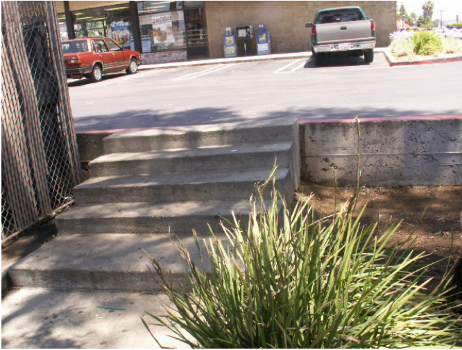
Concrete steps from the finish grade at the Subject Property connect to the property at the north. Note the lack of a handrail.
