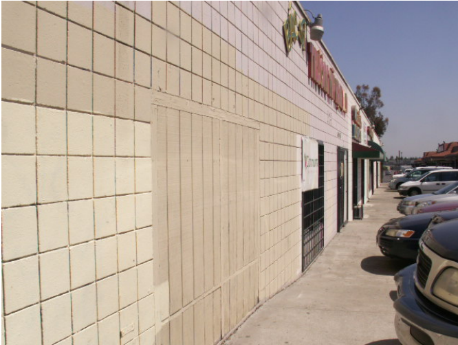
The concrete block wall at the east side of the Building has different colors of paint.
