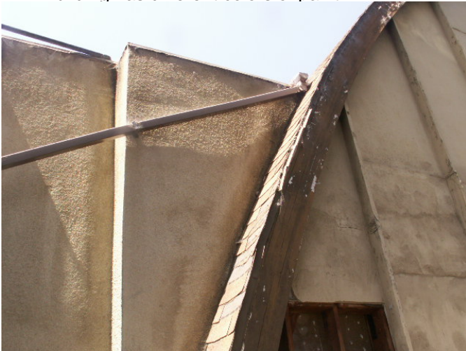
Outside detail of the arched glue-lams on the north side of the Building.
