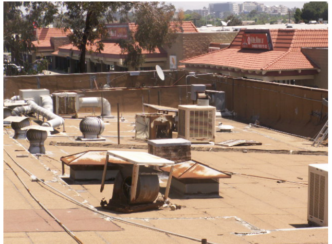
View of the mechanical equipment over the east side of the Building.
