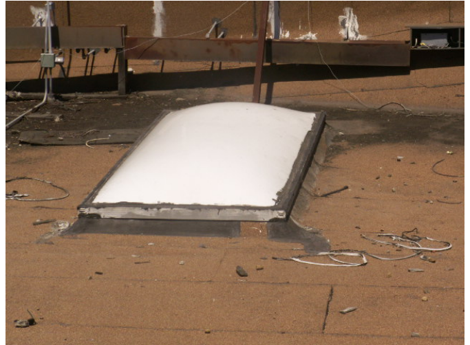
View of the Plexiglas skylight from the roof.
