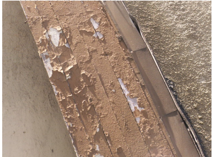
Detail of the glue-lam. Note the need for paint.
