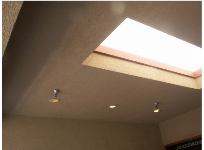
A Plexiglas skylight illuminates the outside entry to the skating rink.
