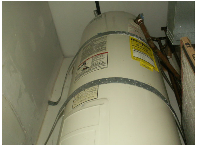
View of a water heater in the medical office.
