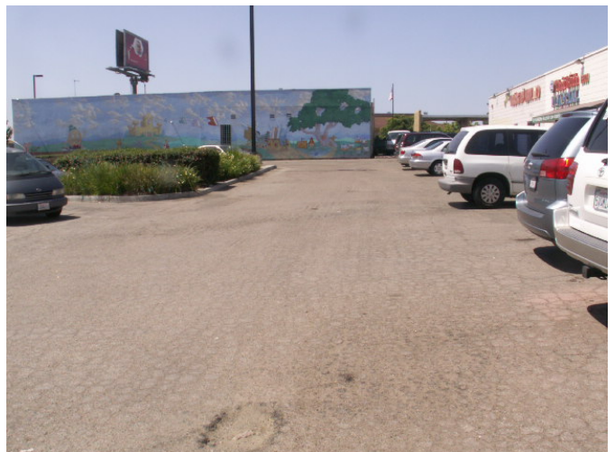
View of the west side asphalt paving. Note pothole in foreground.
