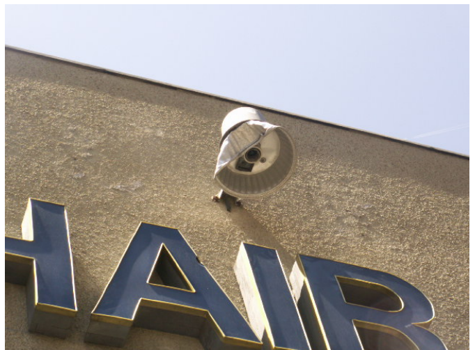
A typical scone lamp requires repair/replacement.
