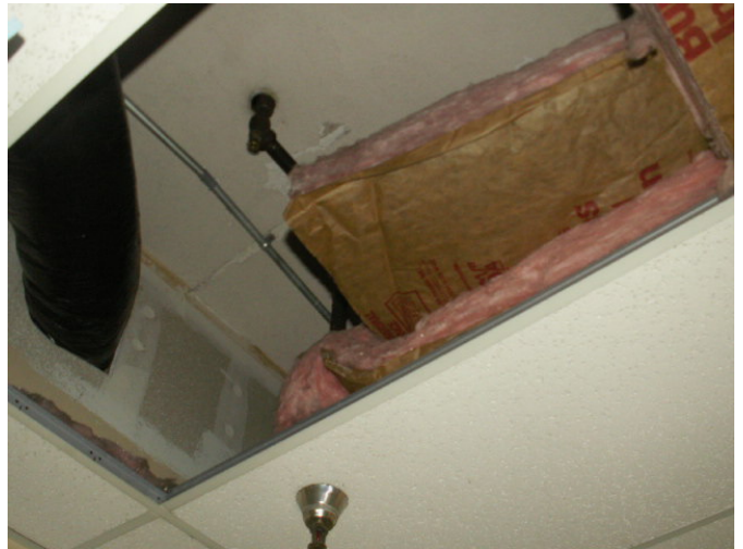
Typical view above the drop-down ceiling at the addition.
