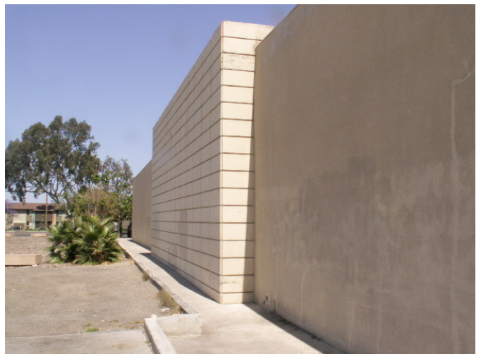
View of the south side of the Building looking west.
