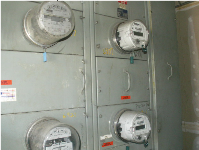
Tenants are individually metered for electricity.
