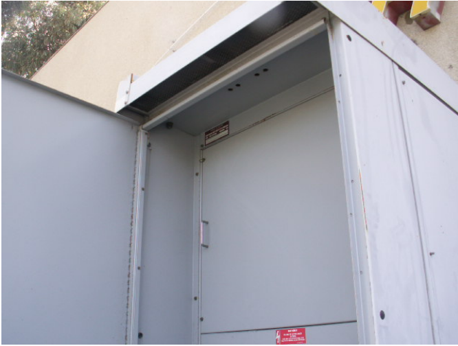
A metal electrical cabinet is located on the west side of the Subject Property
