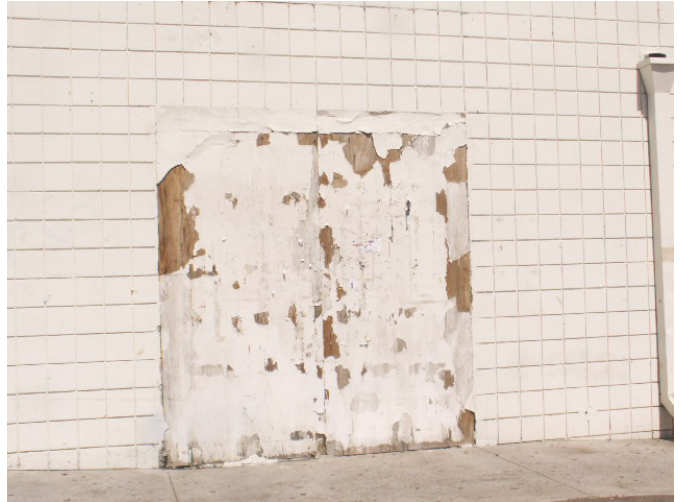
Tenants have enclosed openings as windows and doors have been relocated.
