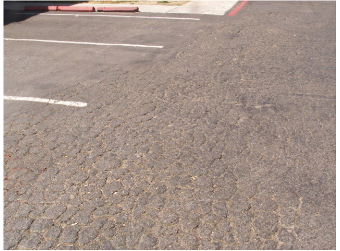
The asphalt is alligator at the west parking lot.
