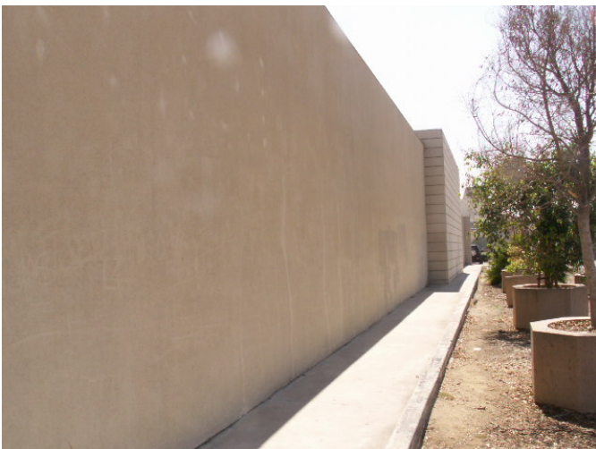
View of the south side of the Building looking east.
