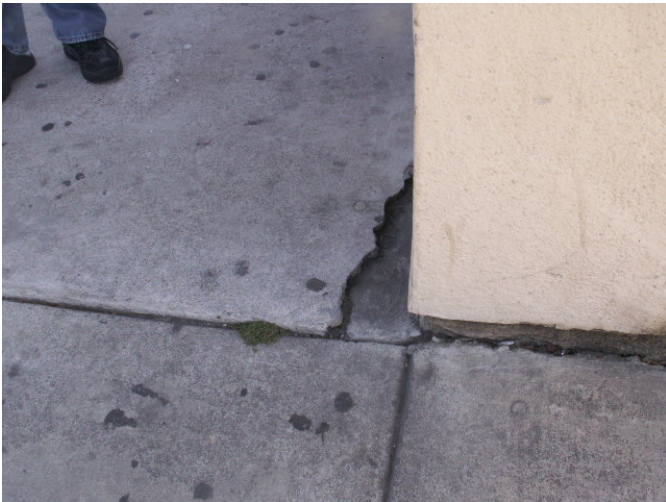
Uneven pavement at the southwest corner of the Building.
