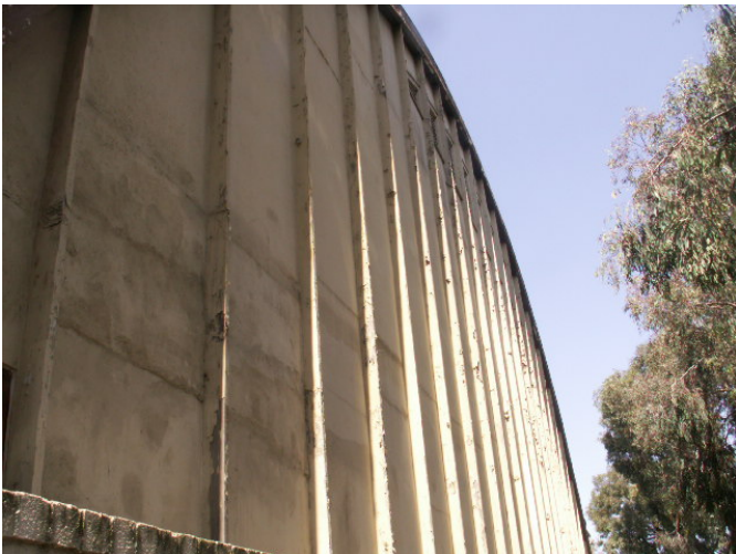
North side elevation at the skating rink. Note the top of the glue-laminated beam/girder arch.
