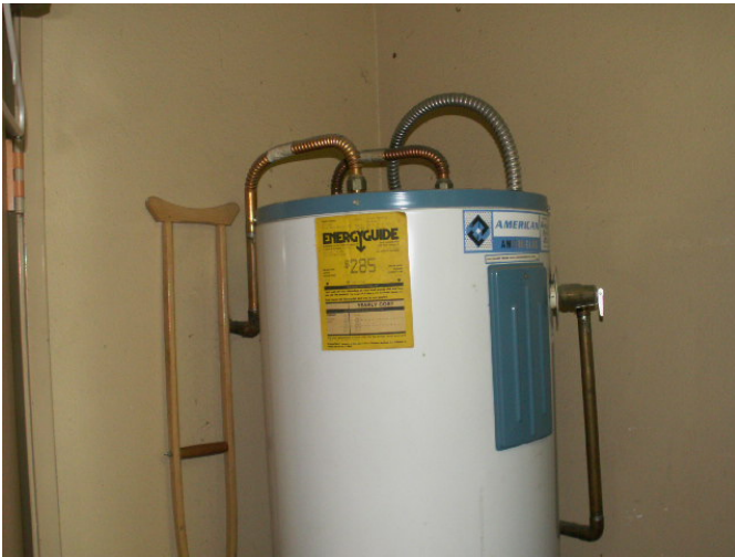
View of a typical electric water heater in one of the tenant spaces.
