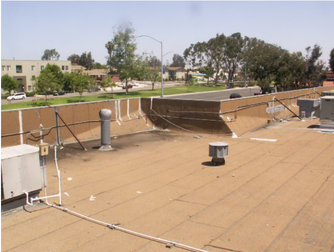
View of the flat roof at the west side of the Subject Property looking northwest.
