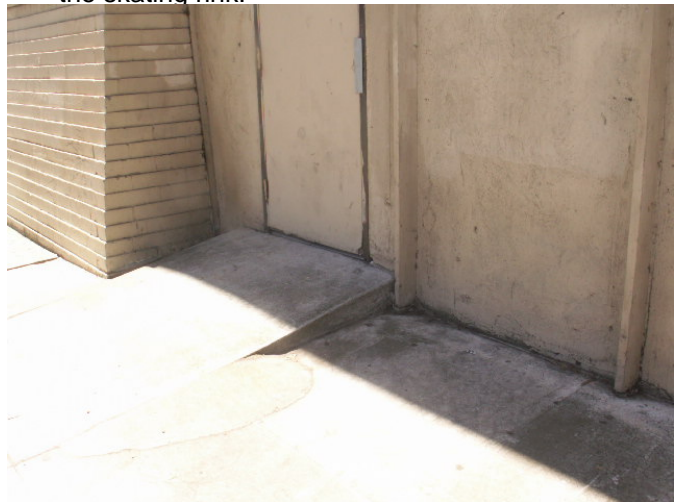
A concrete ramp has been installed from the concrete walkway at the north side of the Subject Property to a door at the skating rink.
