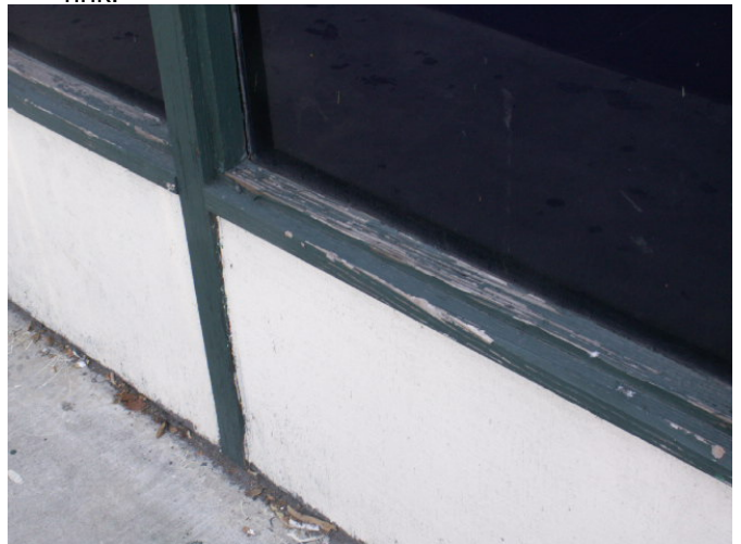
The paint around the windows is flaking.
