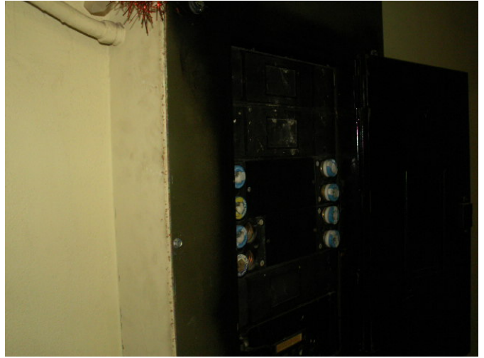
The mezzanine over the skating rink has a fuse box that is connected to the main circuit breaker.
