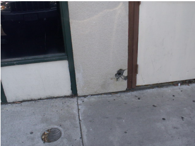
A hole was observed at the base of the stucco on the west side of the Building.
