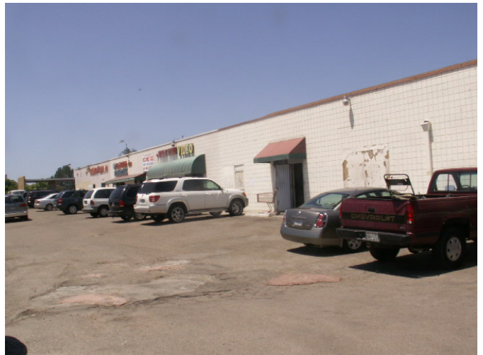
East side elevation looking south.
