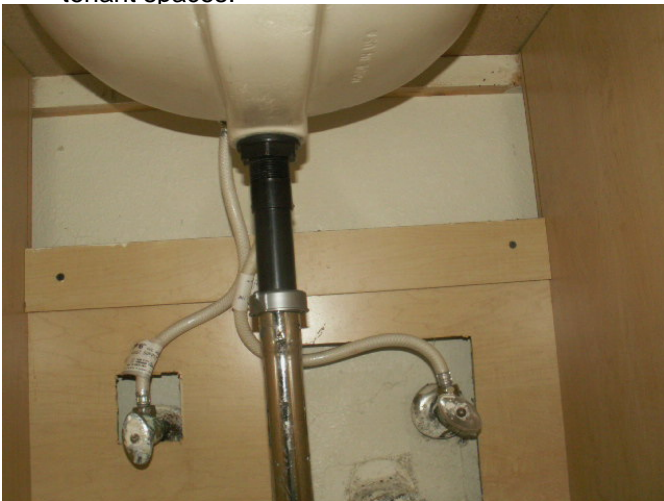
View under a typical sink.
