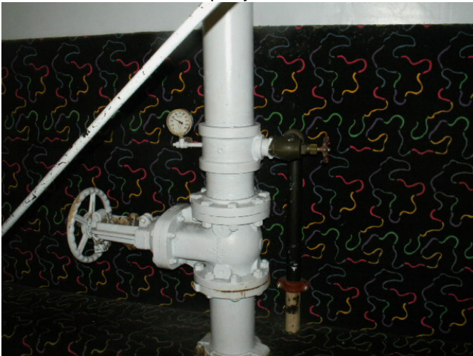
This is representative picture of a wet-system fire sprinkler riser.
