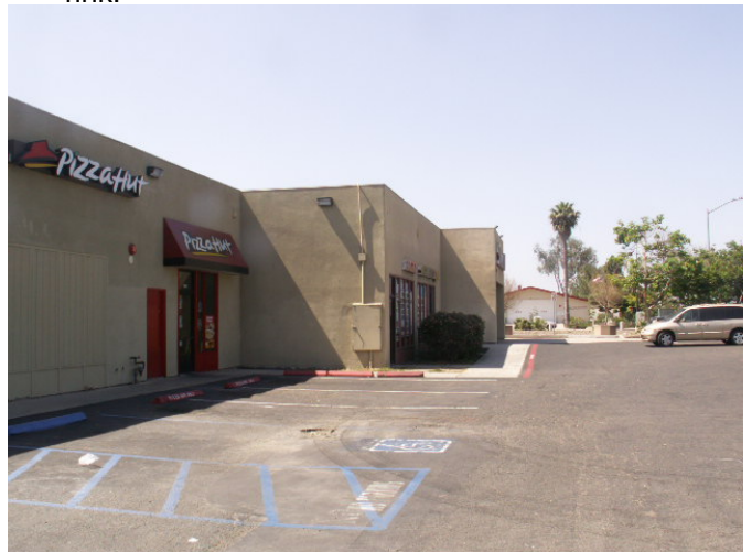
West side of the Building looking south.
