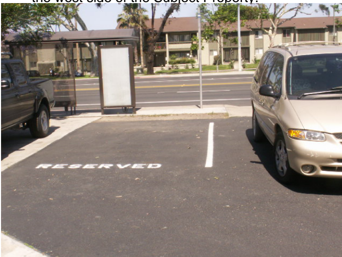
Parts of the asphalt paving are in good condition.
