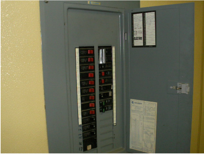
The Subject Property is protected from electrical overload by a circuit breaker.
