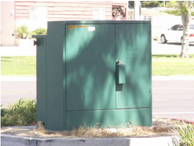
A pad-mounted utility-owned electrical transformer is located adjacent to Linda Vista Road on the west side of the Property.
