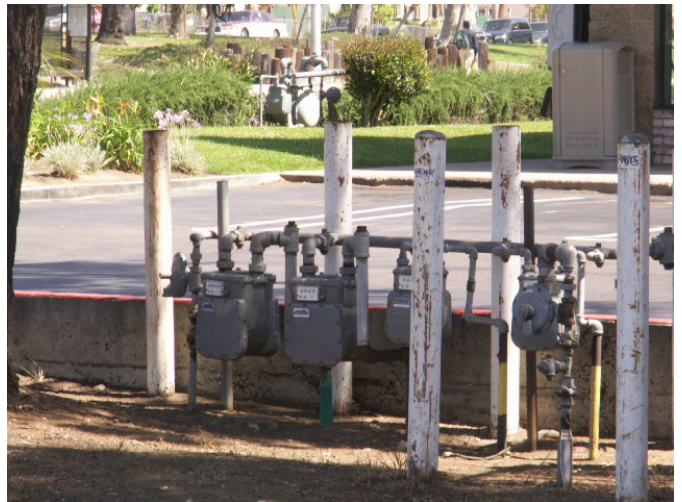
Tenants are individually metered for gas service. Gas meters are located at the north side of the Subject Property.
