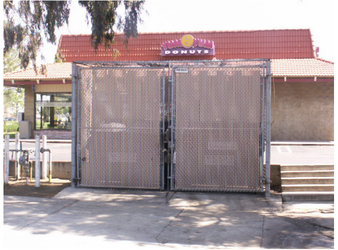
The trash enclosure is located on the north side of the Subject Property and is enclosed in slat-lined chain link.
