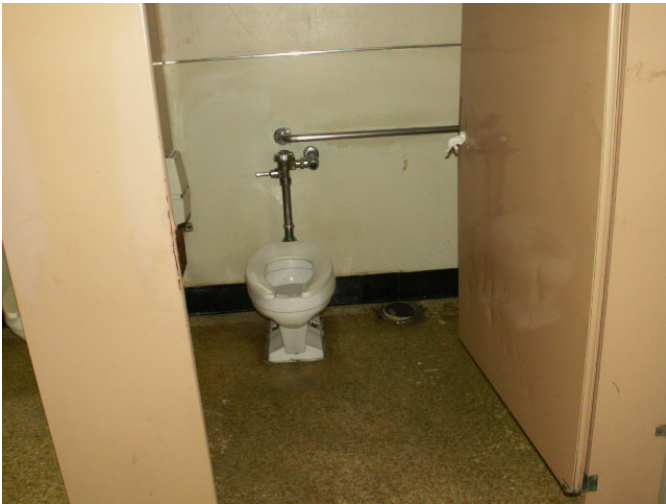
Typical restroom stall.
