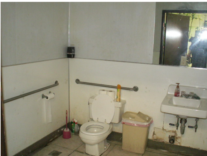
Typical restroom in one of the tenant spaces.
