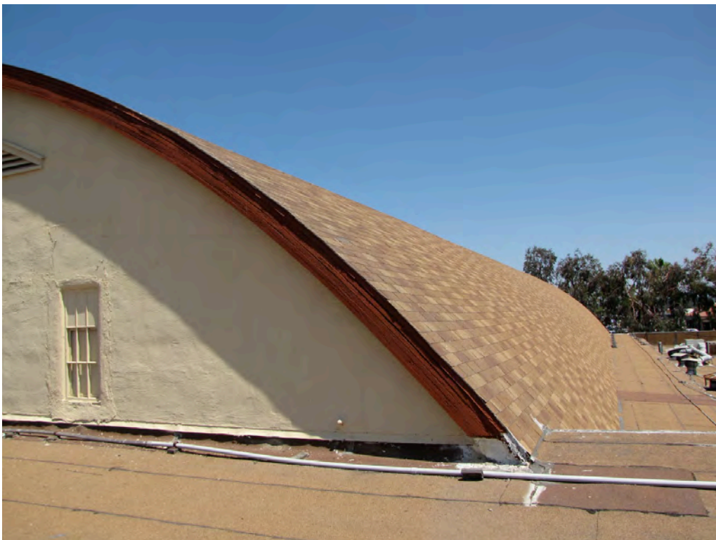
Photo 10: View north of the south ridge of the barrel vaulted roof.
