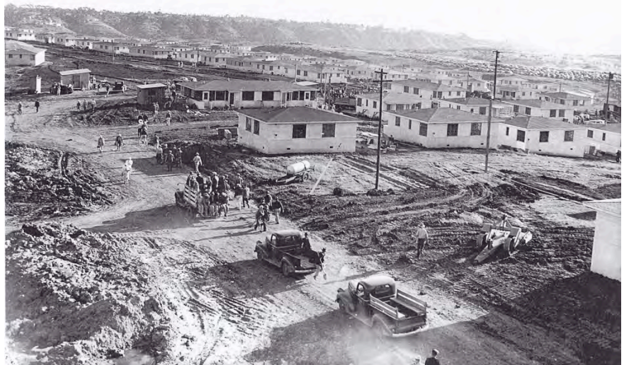
Image 5: Linda Vista Housing Project construction c. 1942-1945. Source: San Diego History Center Photograph Archives.
