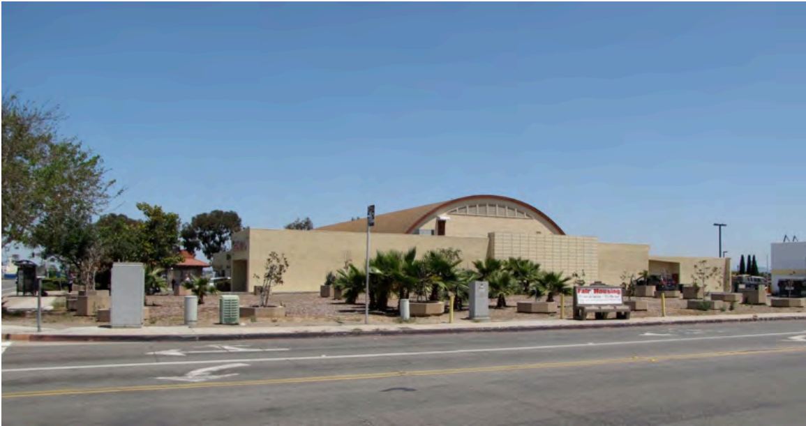
Photo 7: view north of the south elevation showing the extant historic courtyard wall (grid wall) and the original barrel roof with wood slat louvers in the arched gable vent.
