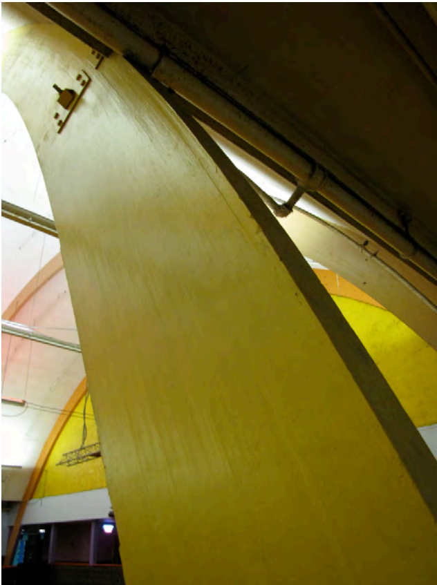
Photo 14: Detail of oversized arched roof truss'
