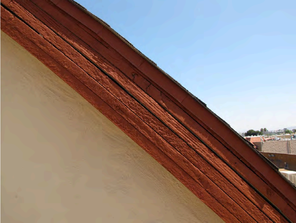
Photo 11: Showing detail of the arched fascia boards that enclose the north and south rooflines.
