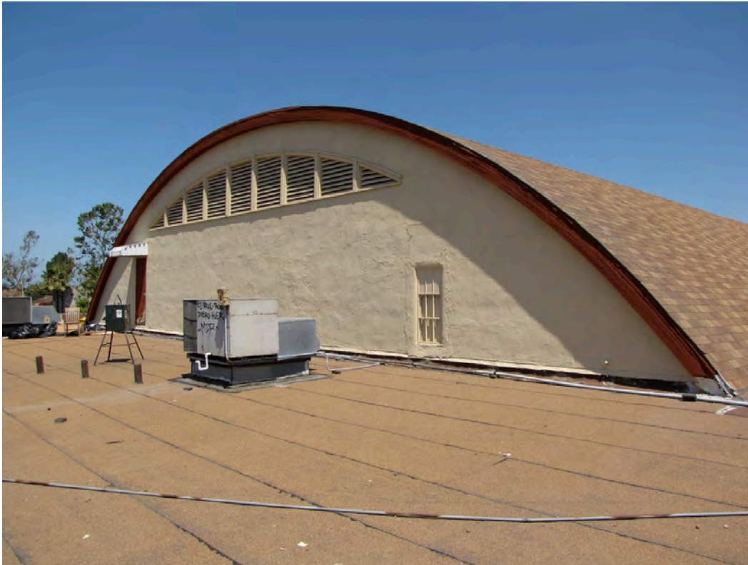
Photo 9: View northwest of the barrel vault roof's south gable wall.
