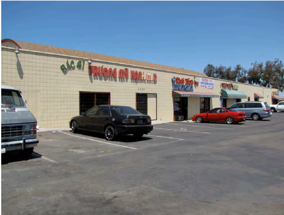
Photo 5: view northwesterly of the east elevation.
