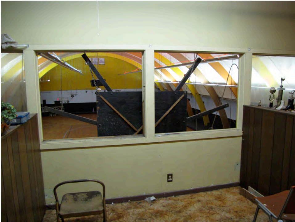
Photo 19: View of the historic truss system from the historic projection room.
