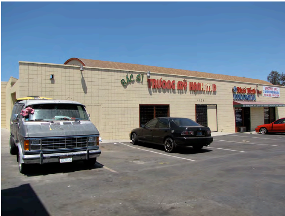
Photo 6: view of the south corner of the east elevation.
