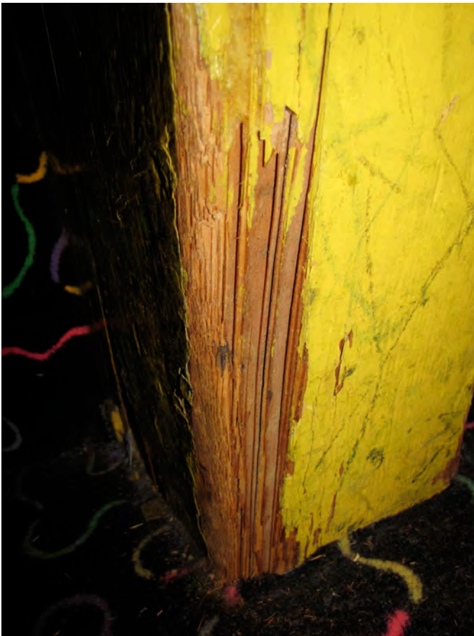
Photo 16: Detail of oversized arched roof truss base and wood exposure.
