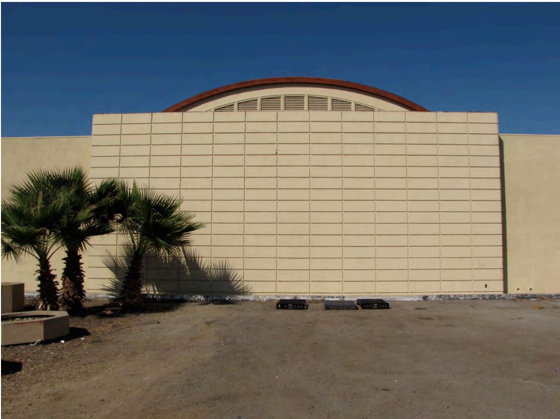
Photo 8: Detail view of extant historic courtyard wall (grid wall).
