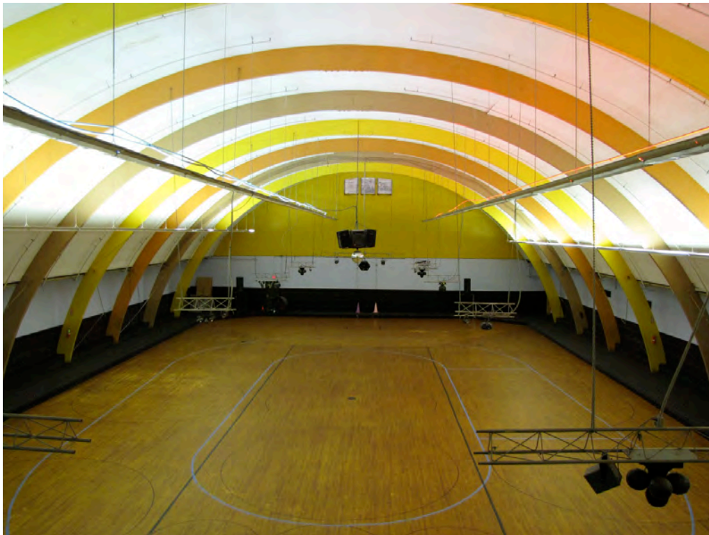
Photo 12: view north of the skate-rink area interior showing oversized arched roof trusses.
