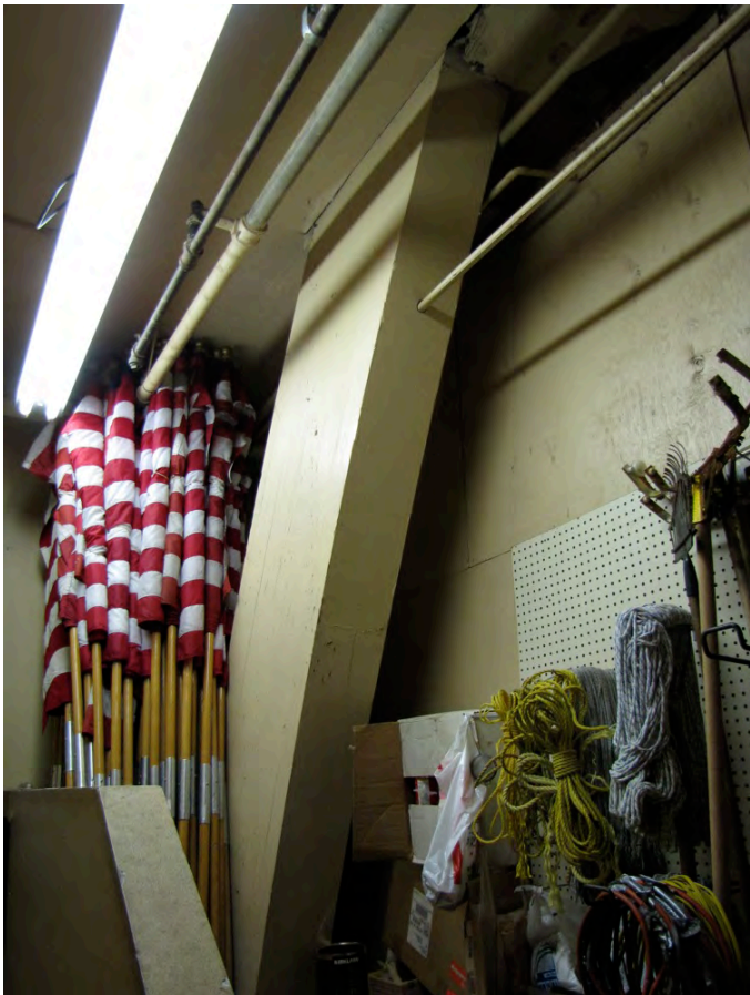
Photo 20: Detail of roof truss spanning through the projection room.
