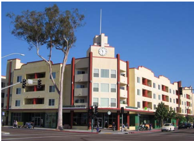
Renaissance at North Park Apartments and Commercial
