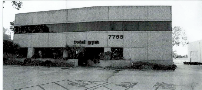
NORTH FACE OF BUILDING
