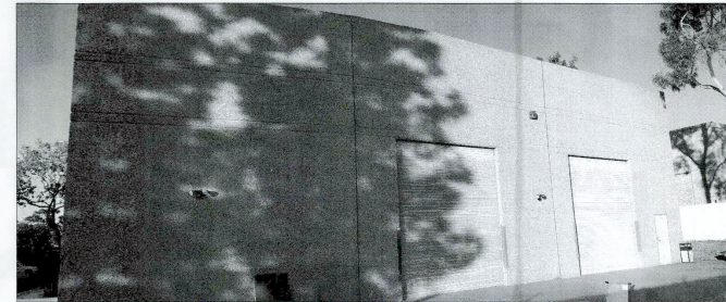
SOUTH FACE OF BUILDING
