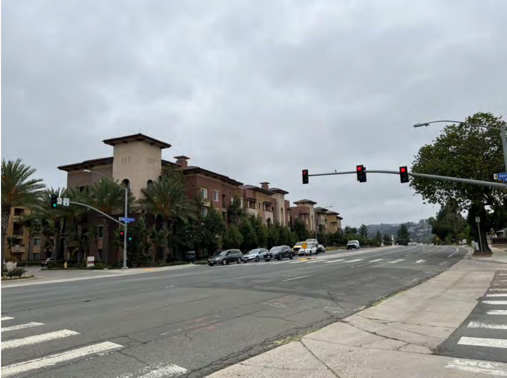
Southeast Elevation @ Greenbriar Ave
