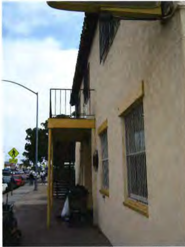
4061 Fairmont Avenue March 2017 Photograph #9 View North of the West façade
