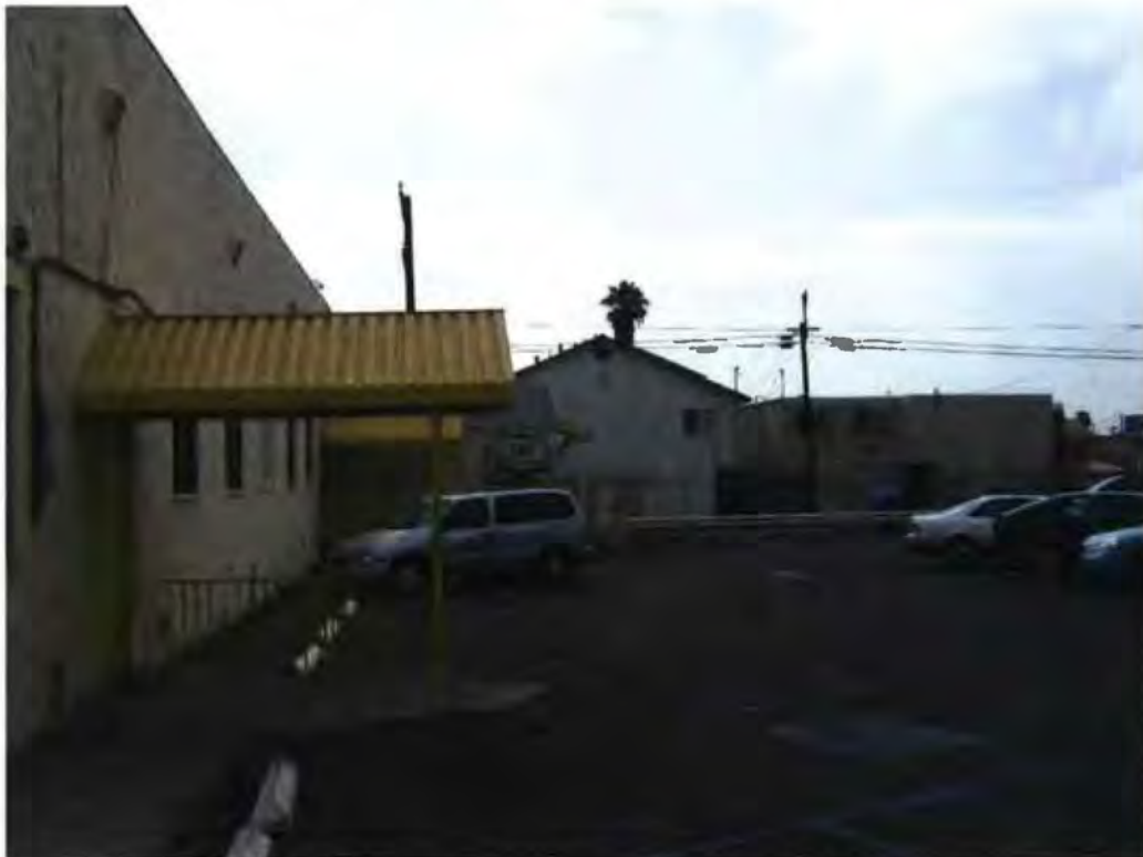
4061 Fairmont Avenue March 2017 Photograph #16 View East of the South façade
