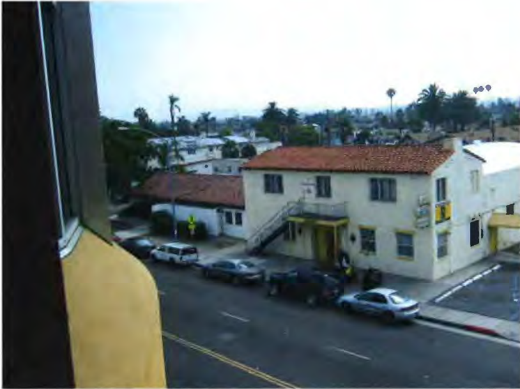
4061 Fairmont Avenue March 2017 Photograph #1 View Northeast of the west façade
