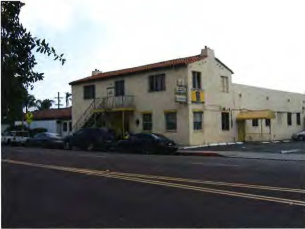
4061 Fairmont Avenue March 2017 Photograph #11 View Northeast of the West and South facades
