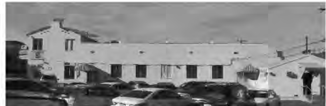
3 PHOTO OF SOUTH ELEVATION 2017 A-1
