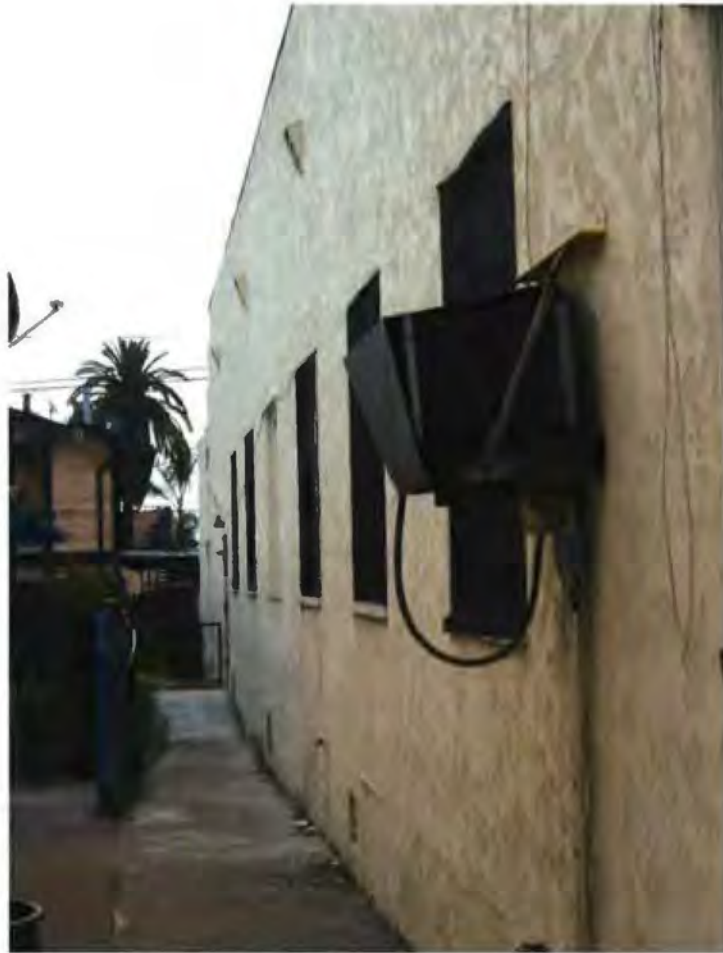
4061 Fairmont Avenue March 2017 Photograph #15 View East of the North façade
