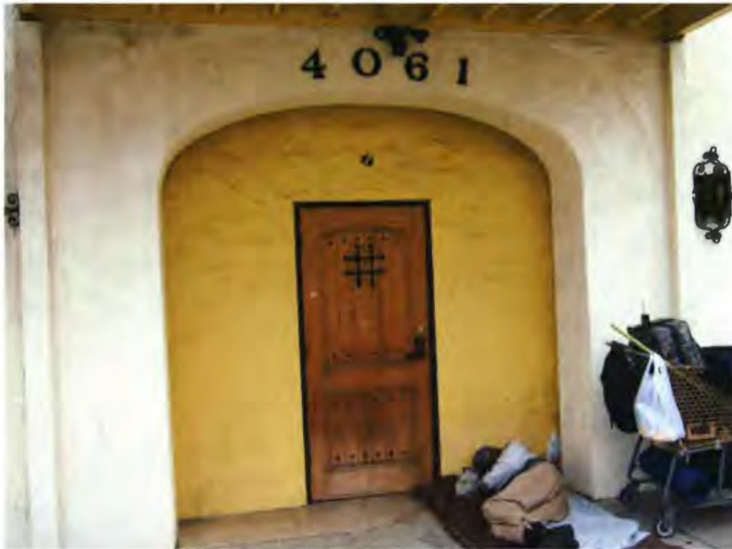
4061 Fairmont Avenue March 2017 Photograph #7 View of main entrance on the West façade
