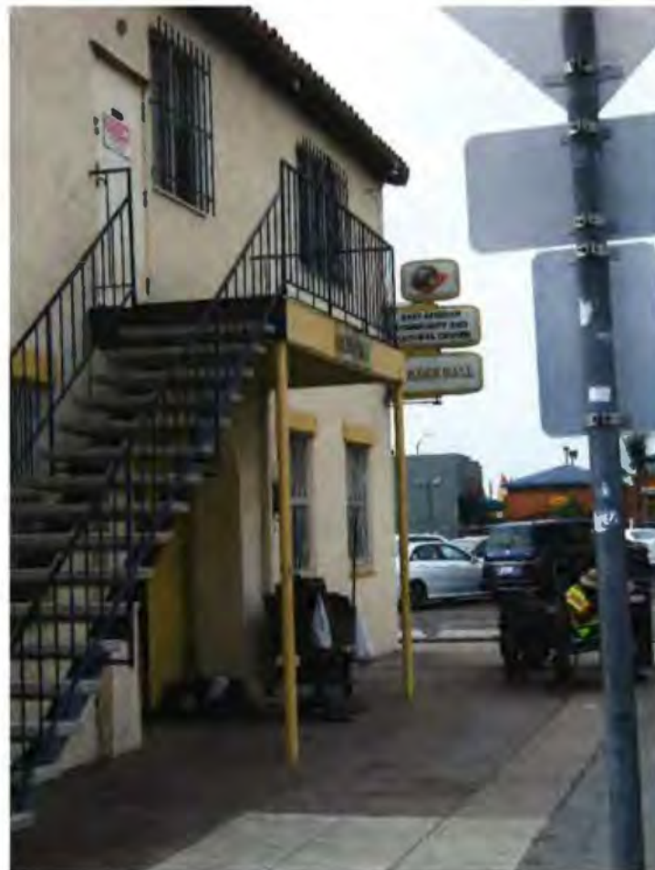
4061 Fairmont Avenue March 2017 Photograph #8 View South of the West façade
