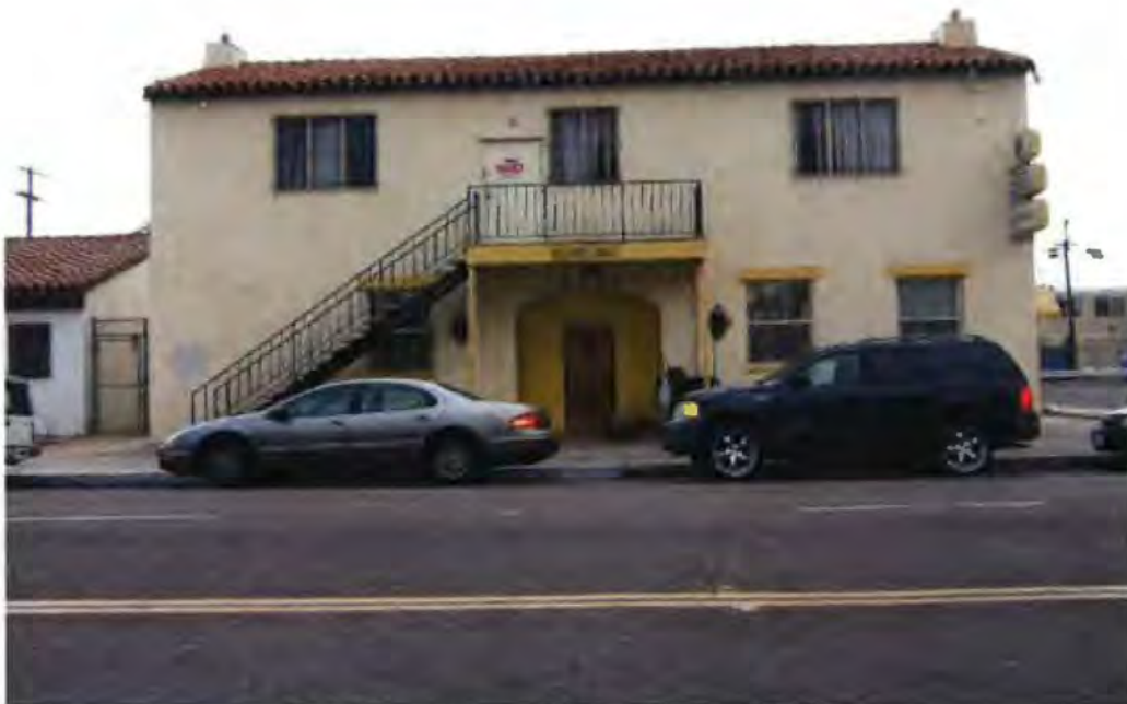
4061 Fairmont Avenue March 2017 Photograph #3 View East of the West façade
