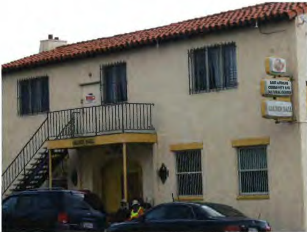
4061 Fairmont Avenue March 2017 Photograph #2 View of the West façade
