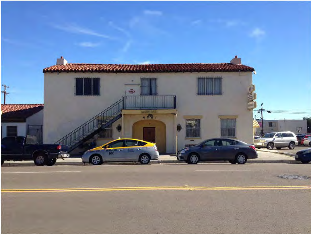
View of 4061 Fairmount Ave looking east towards project site
