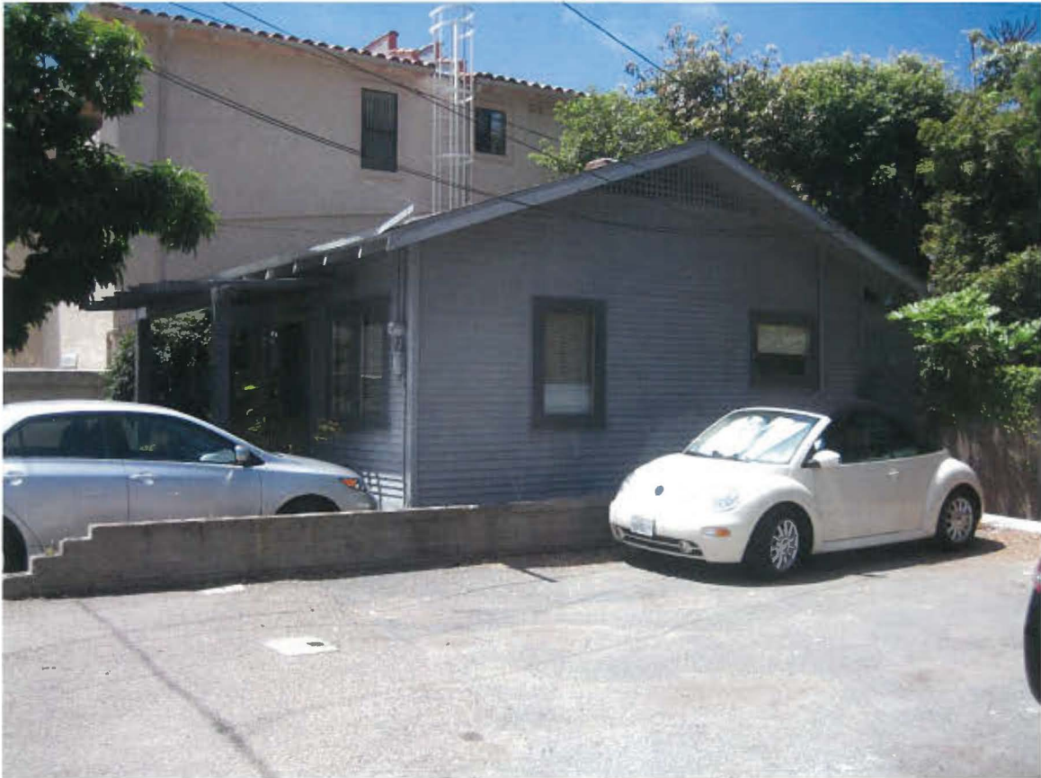
Photograph #6 7762 Bishops Lane East & North Elevations View Facing South
