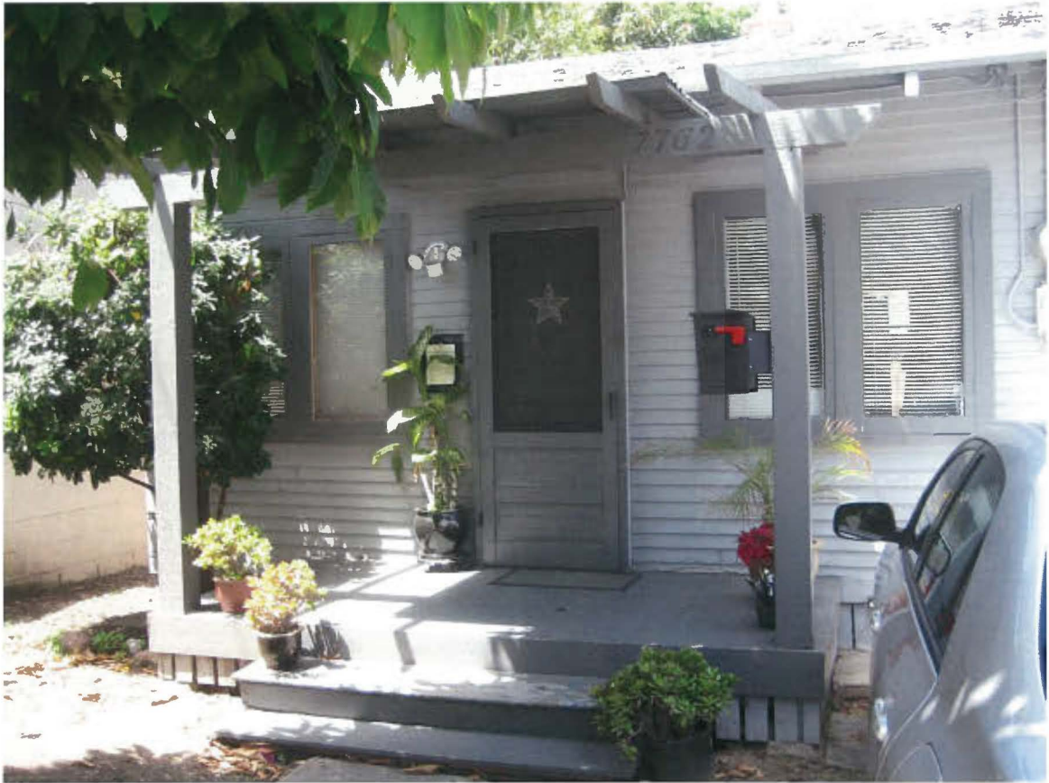
Photograph #7 7762 Bishops Lane East Elevation View Facing West
