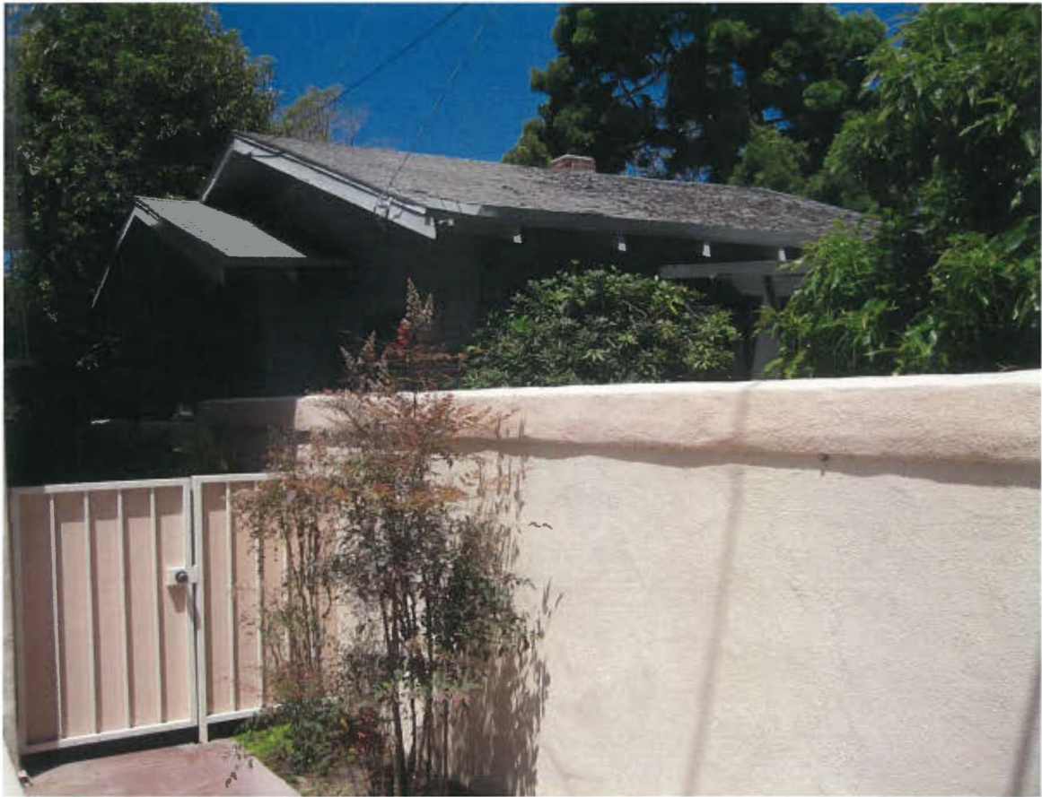
Photograph #9 7762 Bishops Lane East & South Elevations View Facing West
