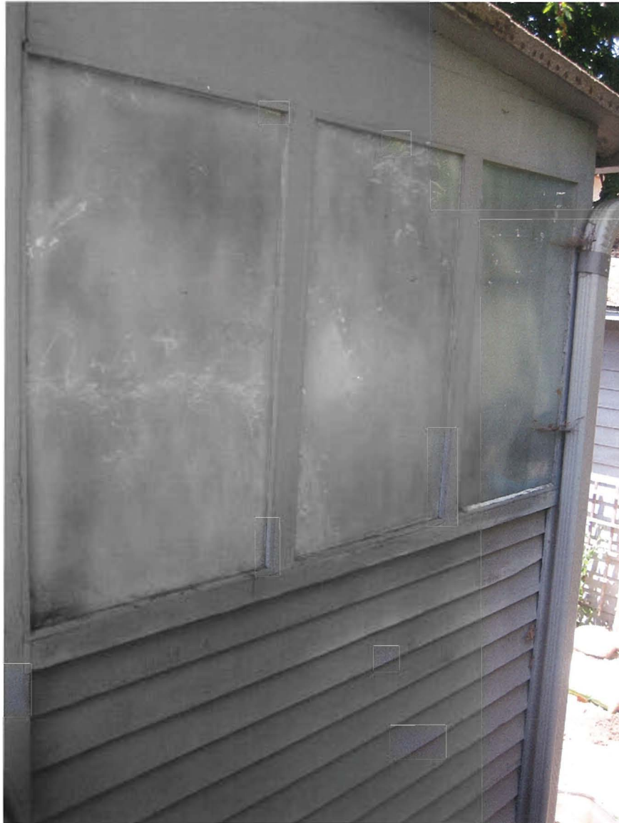
Photograph #11 7762 Bishops Lane Northwest Elevation (Porch Enclosure) View Facing Southwest
