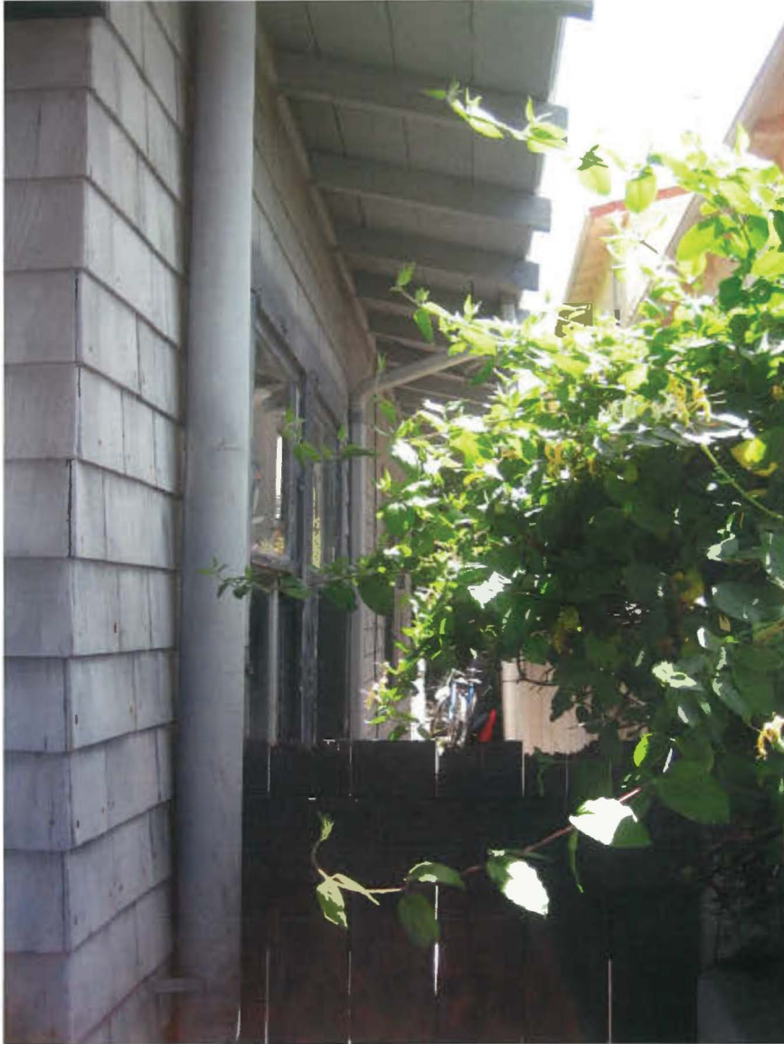
Photograph #4 7761 Eads Avenue South Elevation View Facing East
