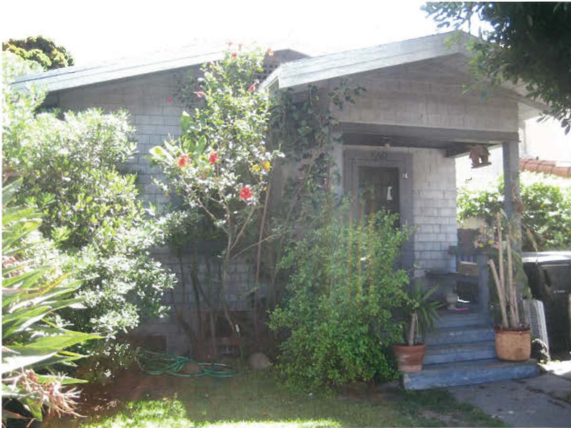
Photograph #2 7761 Eads Avenue West Elevation View Facing East
