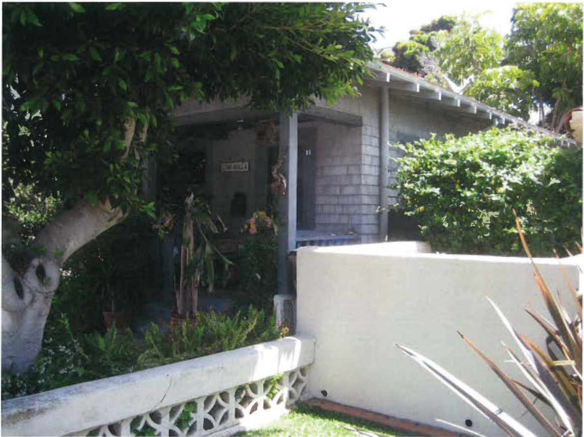
Photograph #3 7761 Eads Avenue West & South Elevations View Facing Northeast
