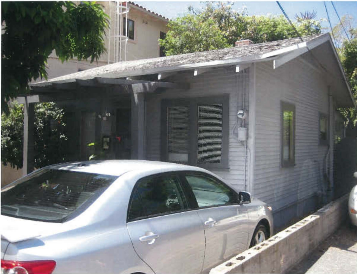
Photograph #5 7762 Bishops Lane East & North Elevations View Facing West
