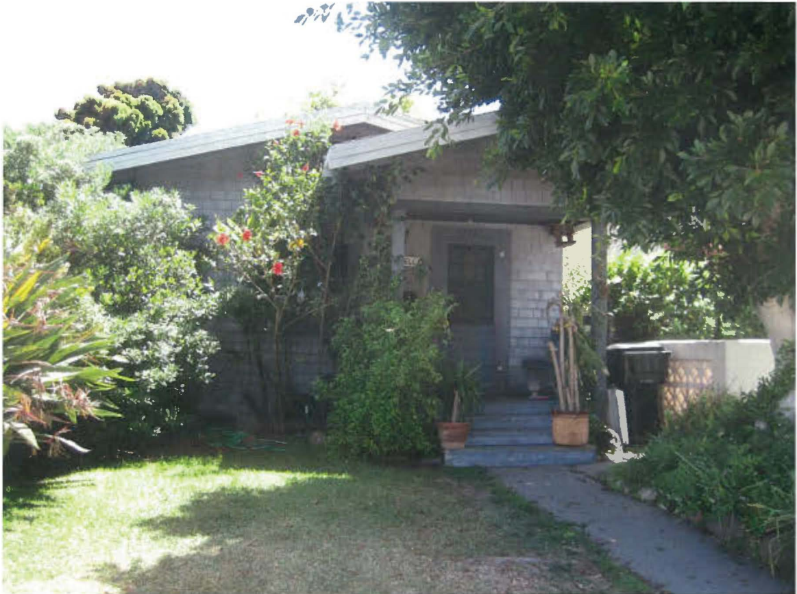
Photograph #1 7761 Eads Avenue West Elevation View Facing East
