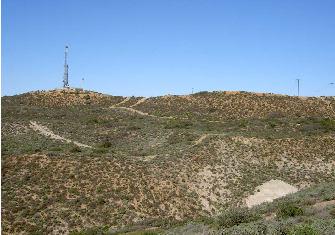
Moody Canyon Landslide – Looking North
