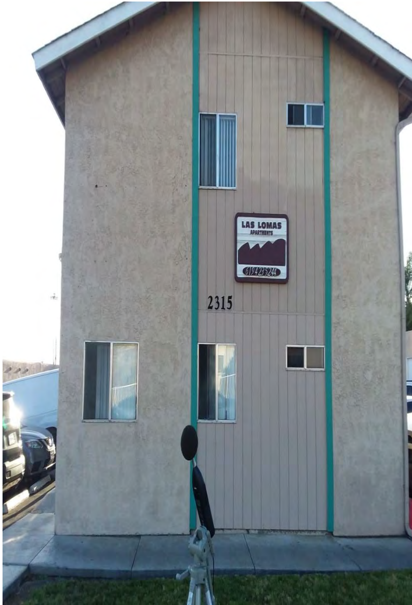
NM11 18 - 03 looking West towards residence.
