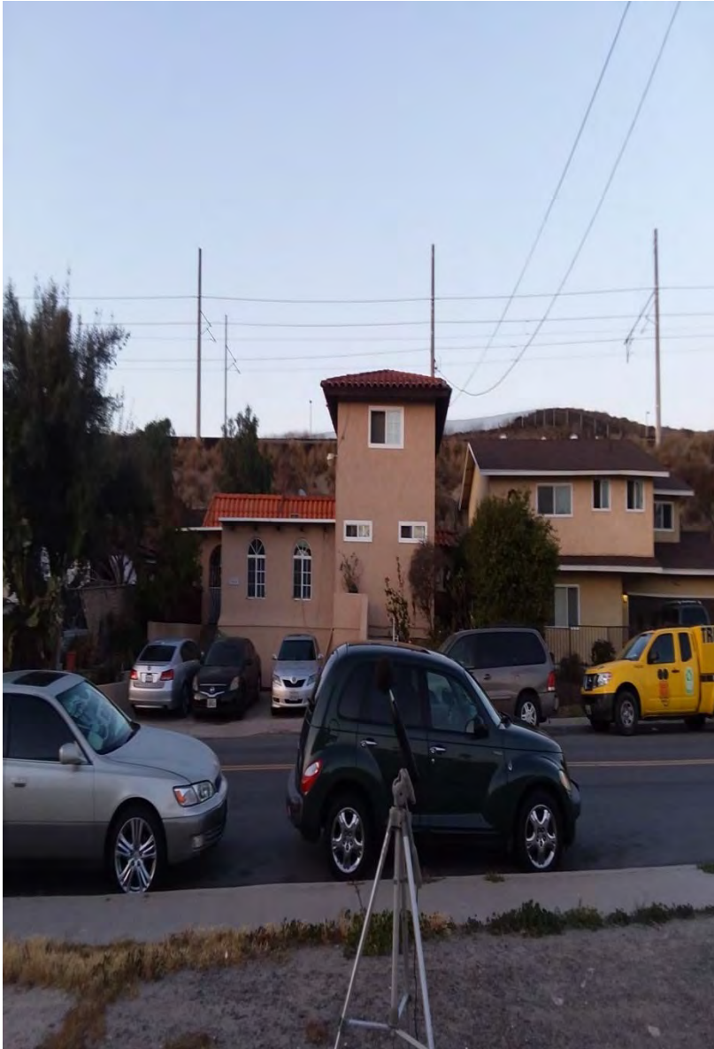
NM13 18 - 03 looking North East towards residence 2641 East Beyer Blvd. Trolley lines run behind residence.
