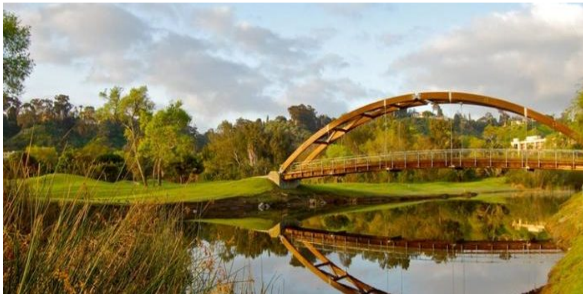
Existing bridge across the San Diego River
