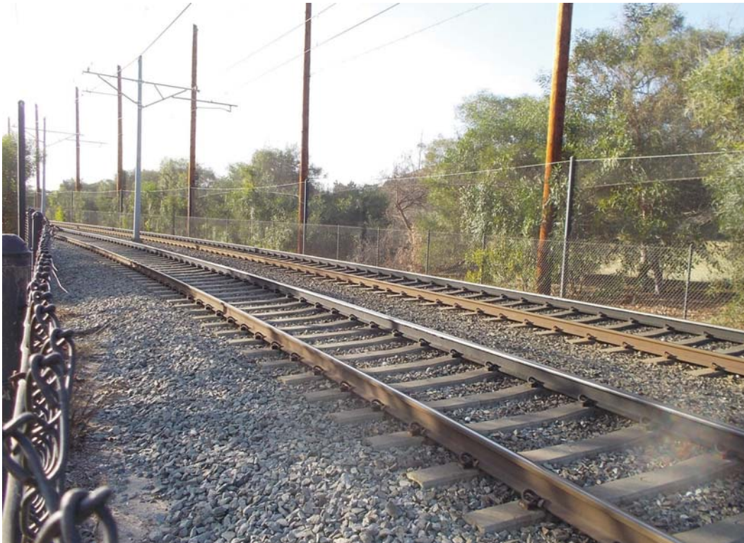
2) View of the MTS trolley line located south of the Site.
