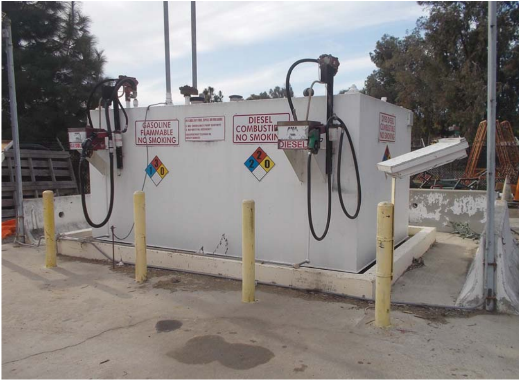
1) View of the gasoline and diesel fuel tank observed on Site.
