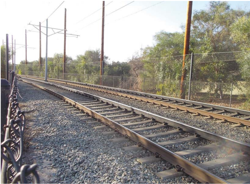
1) View of the MTS trolley line located north of the Site.
