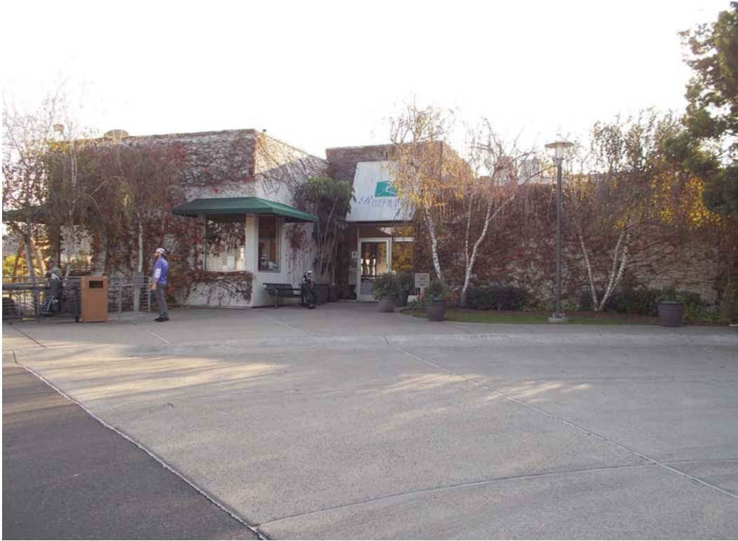
1) View of the Site building looking southeast.
