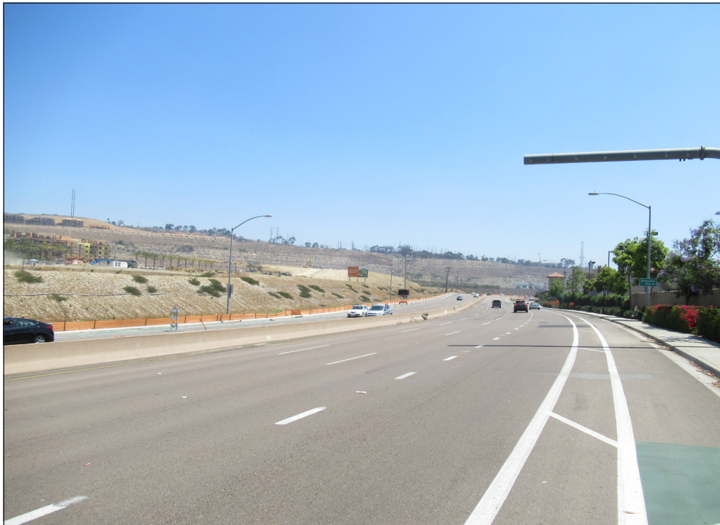
Photo 1. Eastern portion of Friars Road, north of Mission Valley Mall, where the 48-inch water main will be constructed within existing road right-of-way. Looking east.
