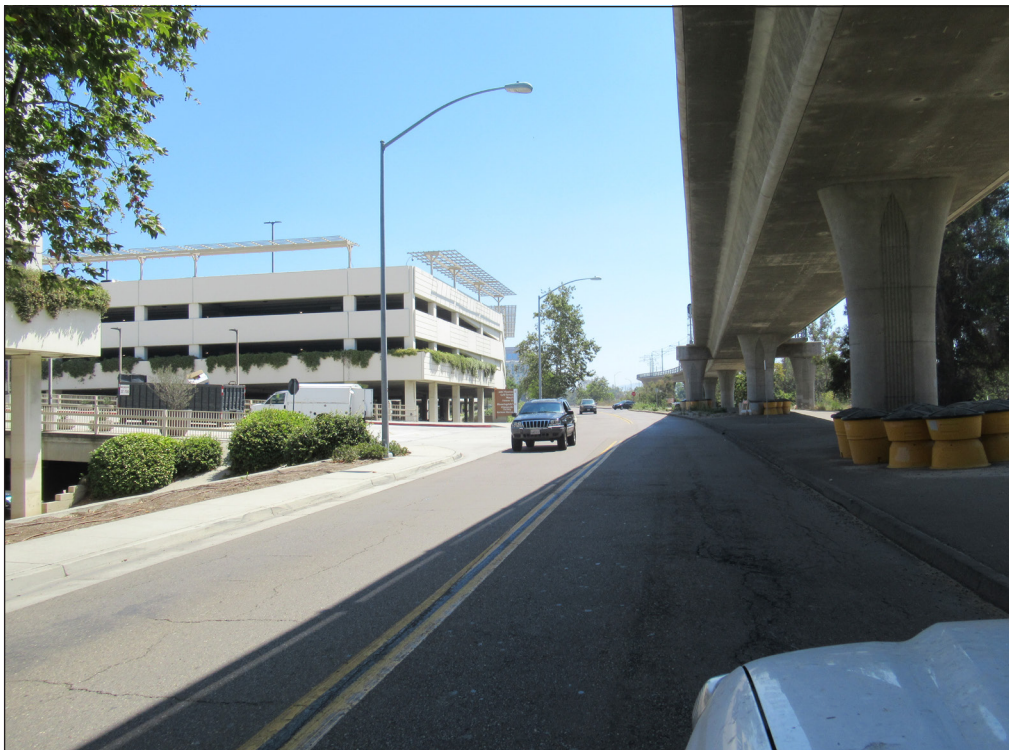
Photo 6. Riverwalk Drive to the south of Fashion Valley Mall where the 48-inch water main will be constructed within the existing road right-of-way. Looking east.
