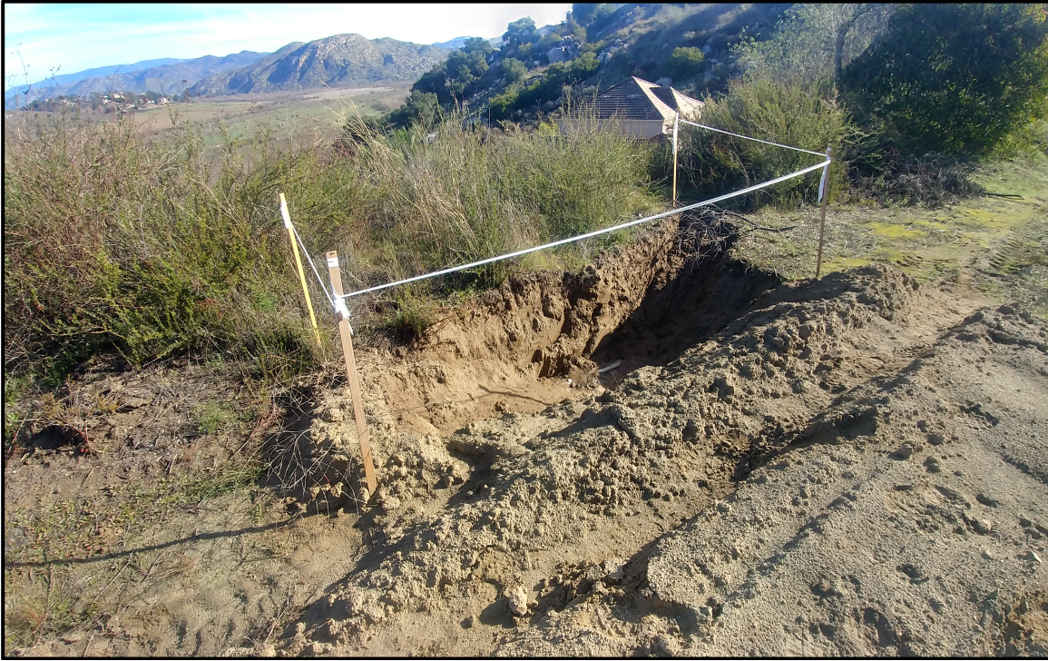
Plate 3: Overview of excavated trench, looking east.
