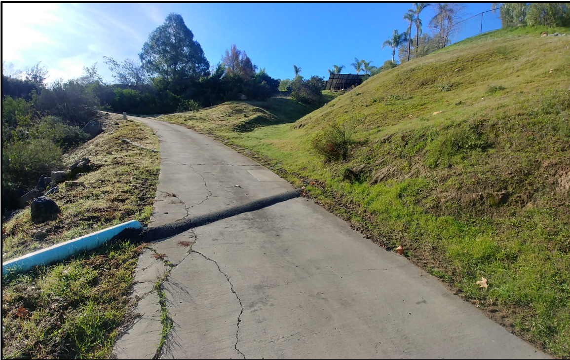
Plate 2: Overview of concrete driveway, looking southeast.
