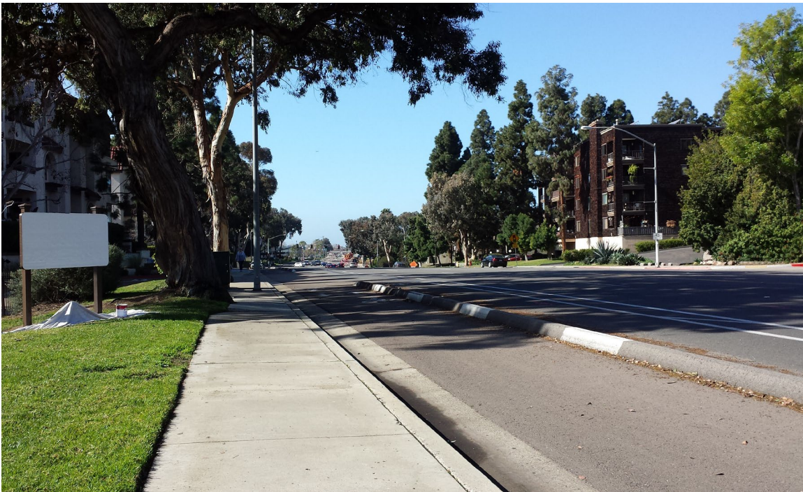
Plate 1. Overview of project alignment along Friars Road, near Colusa Street; view to the west.
