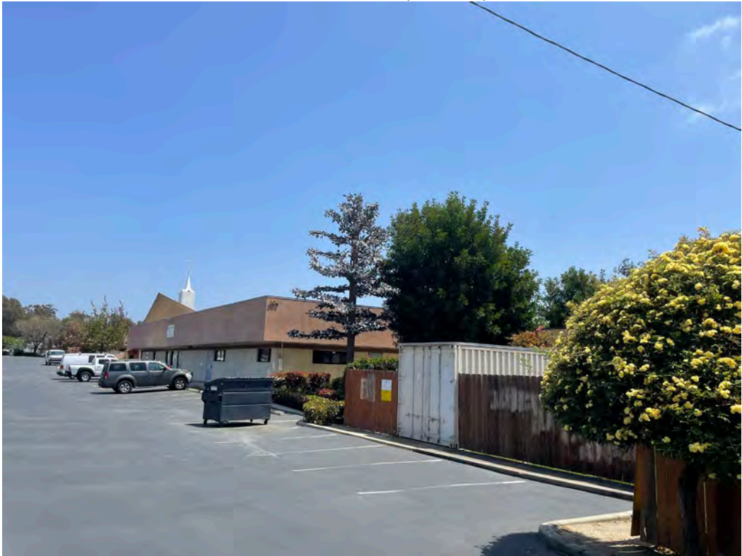
West Elevation (Photo 4)
