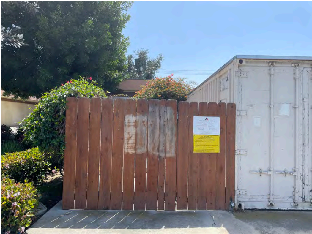
Existing Equipment Enclosure
