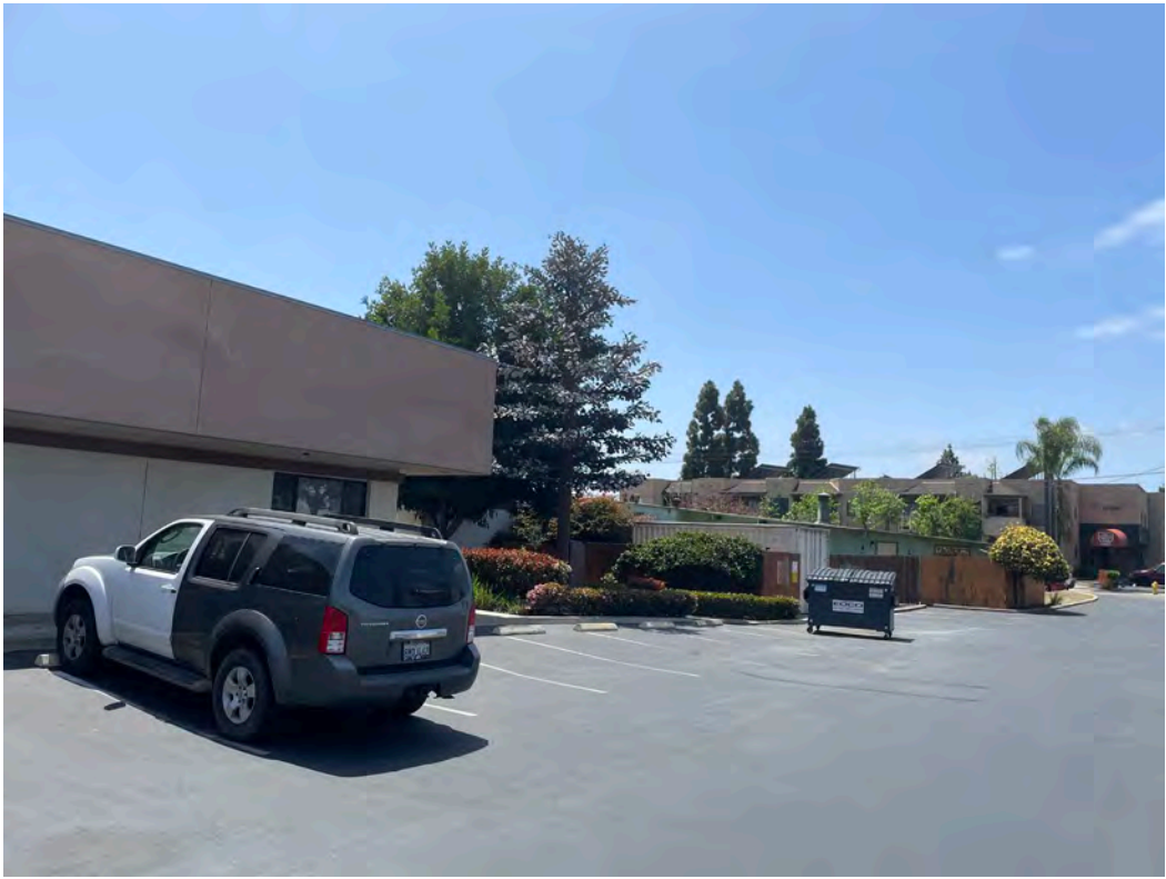
East Elevation (Photo 1)
