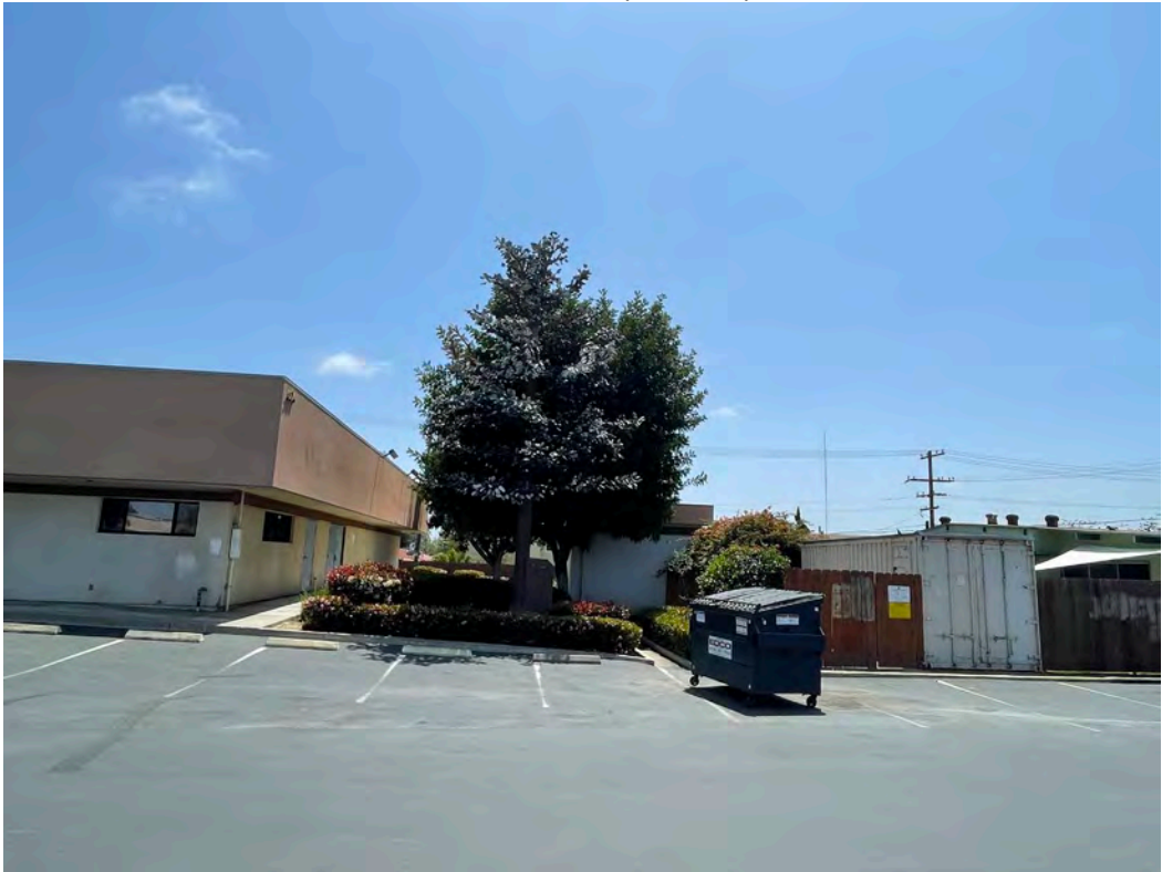
North Elevation (Photo 2)
