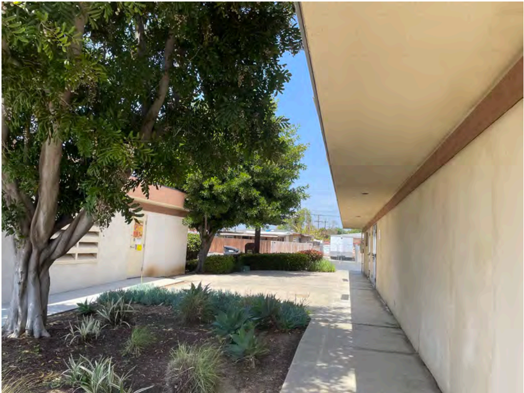
South Elevation (Photo 3)
