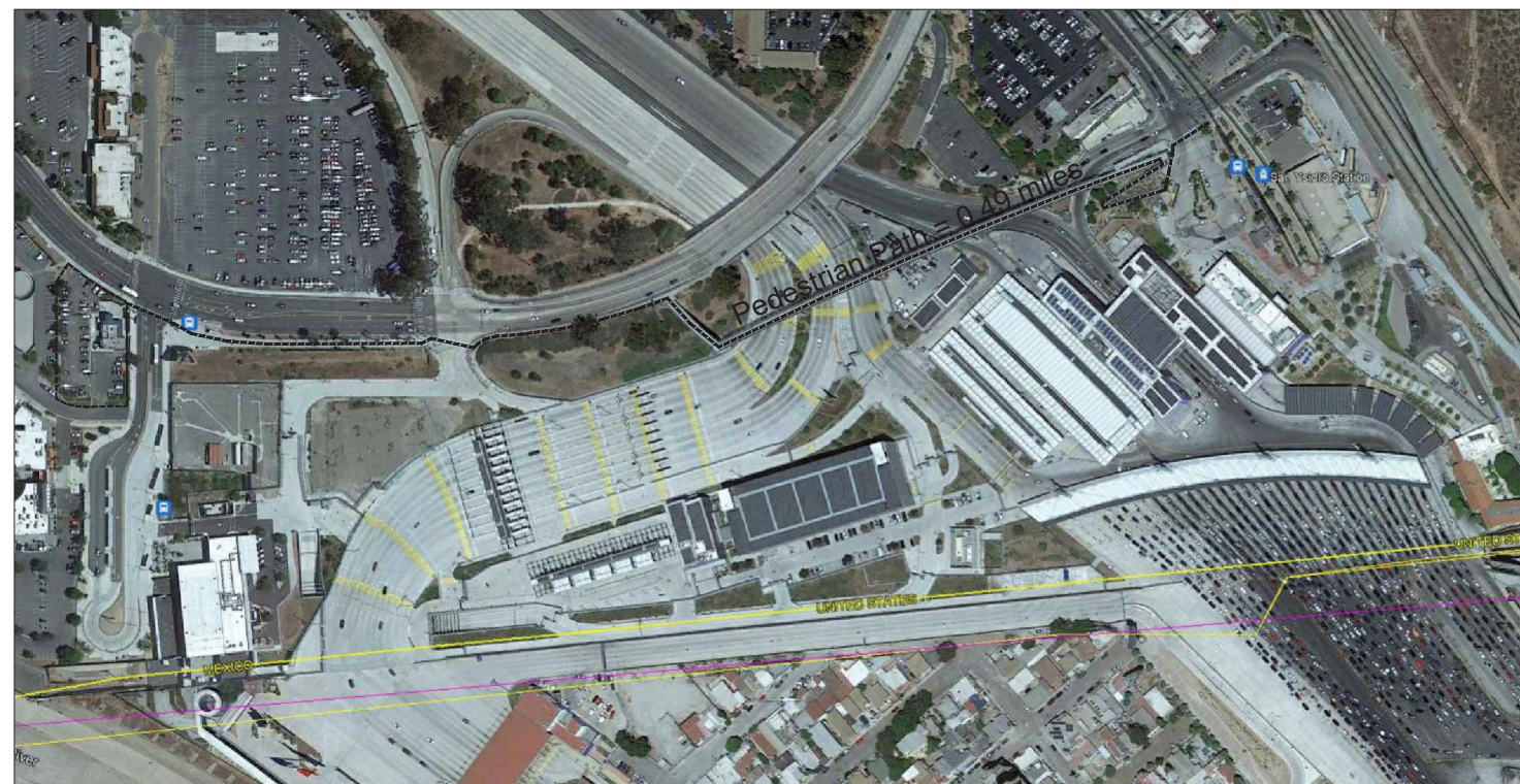
11. Pedestrian Path from Development Project to Existing Passenger Rail Station (San Ysidro Station)
