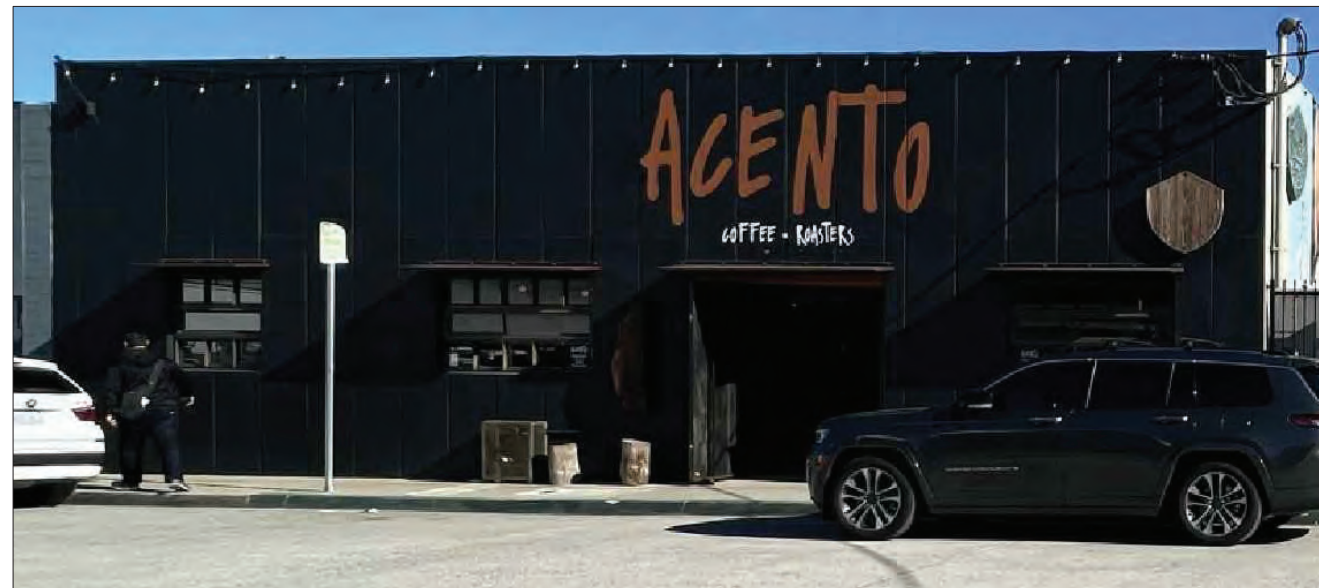
7. Image of Existing West Elevation
