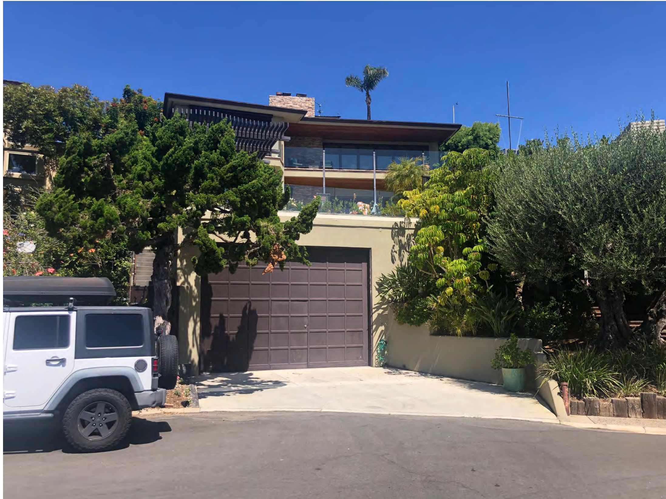
Houses Along San Antonio Place (Public Road) 3 Levels
