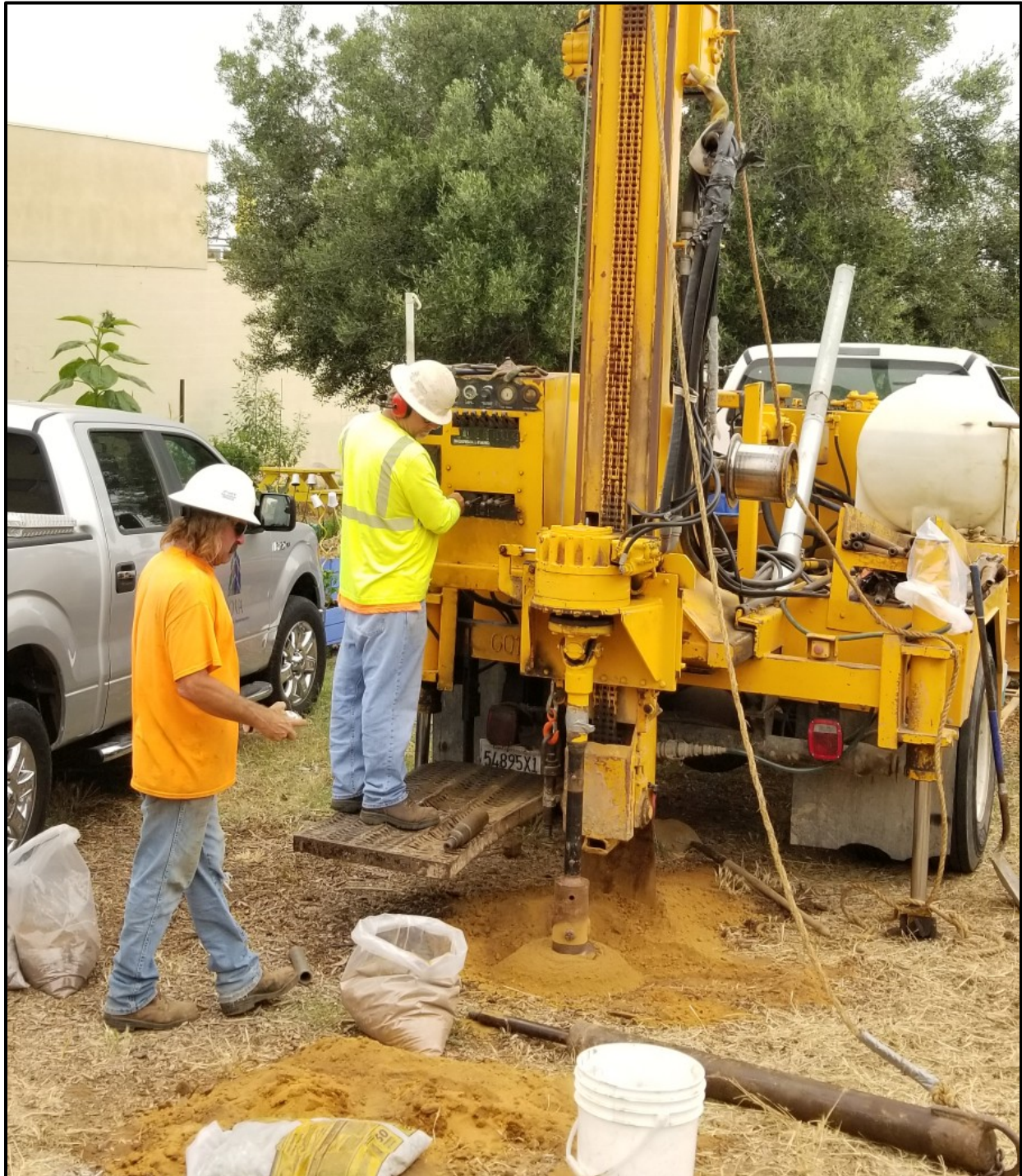
Figure 3-2. Drilling Operations, July 11, 2019
