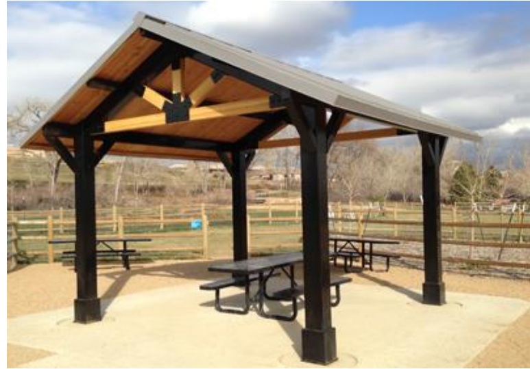
SHADE STRUCTURE WITH COVERED ROOF
